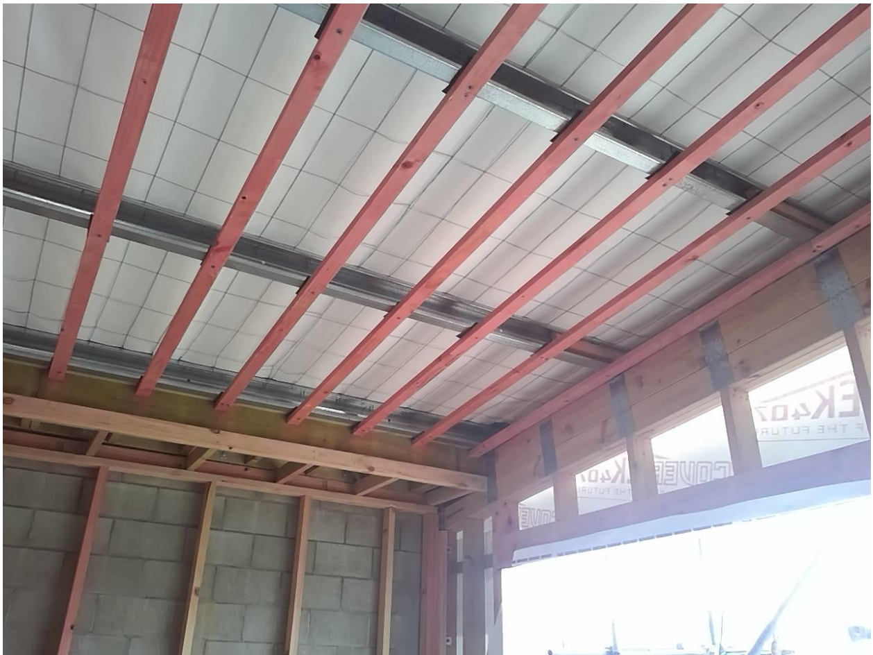
Sample of ceiling battens Taken at 1:35 PM on Wednesday 25/09/2019
