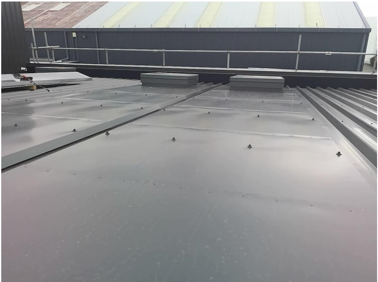
Apron flashings to velux windows on roof. Taken at 1:25 PM on Wednesday 25/09/2019
