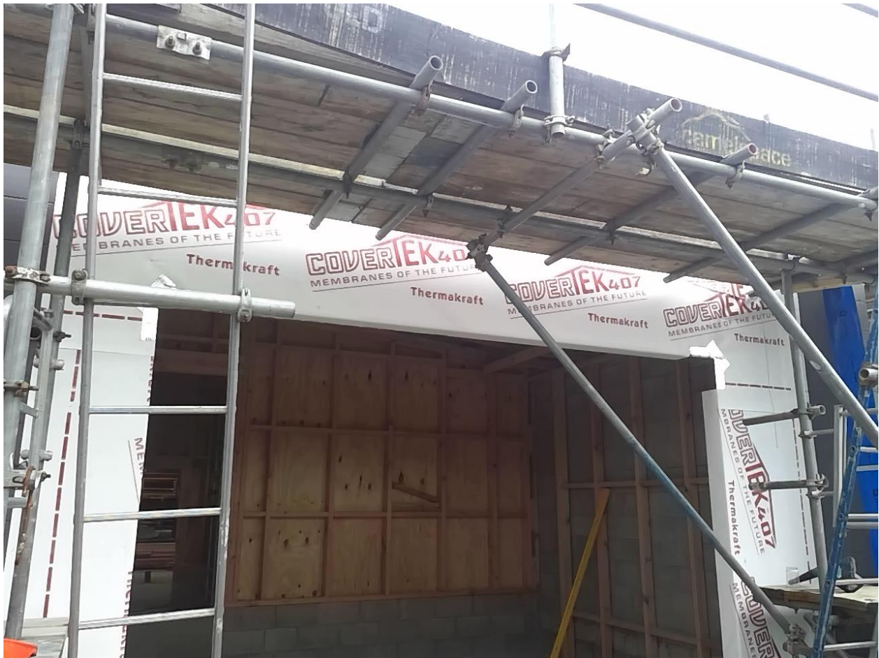
Building wrap to north face Taken at 1:32 PM on Wednesday 25/09/2019
