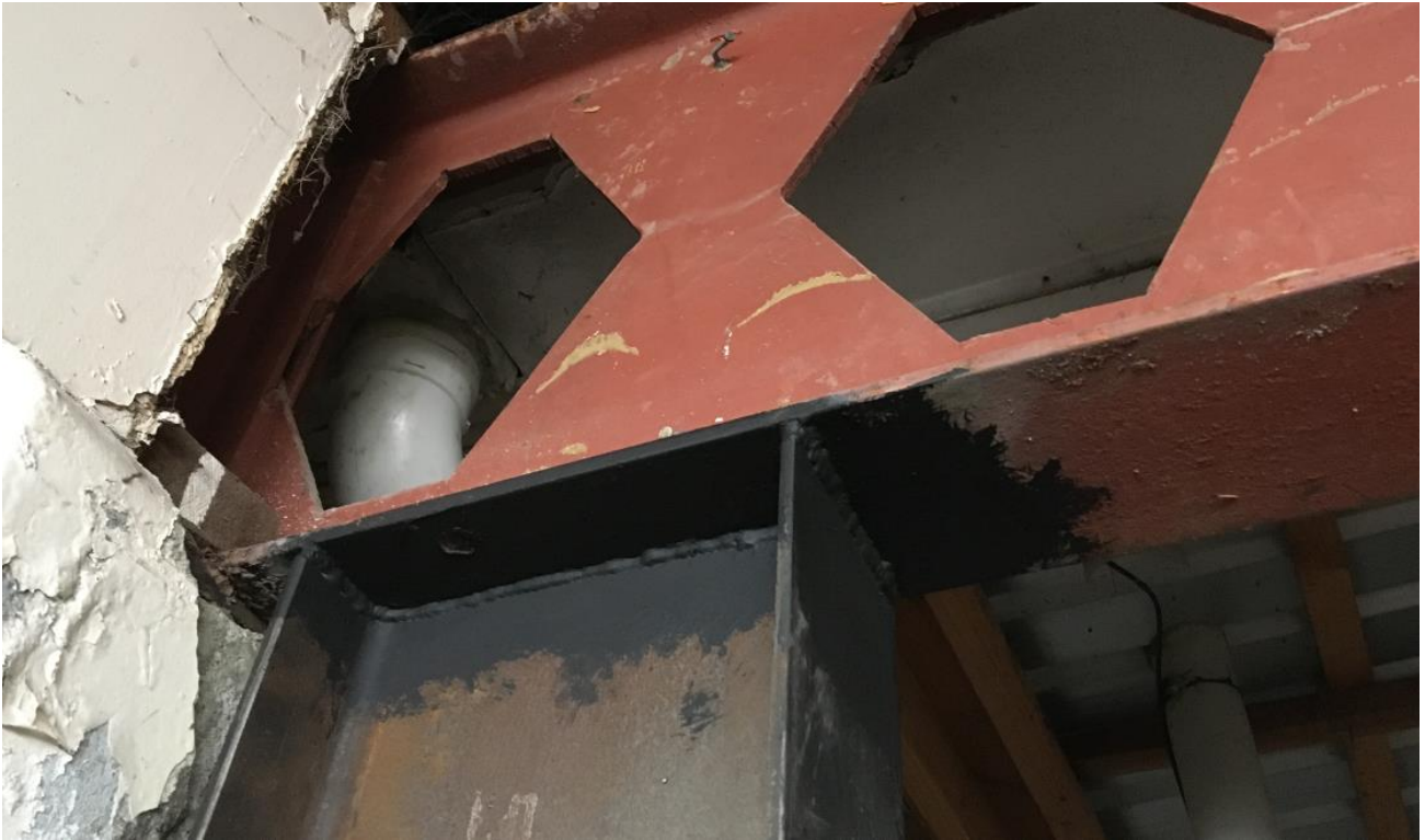
Photo 6 – Column C-3. Top connection
