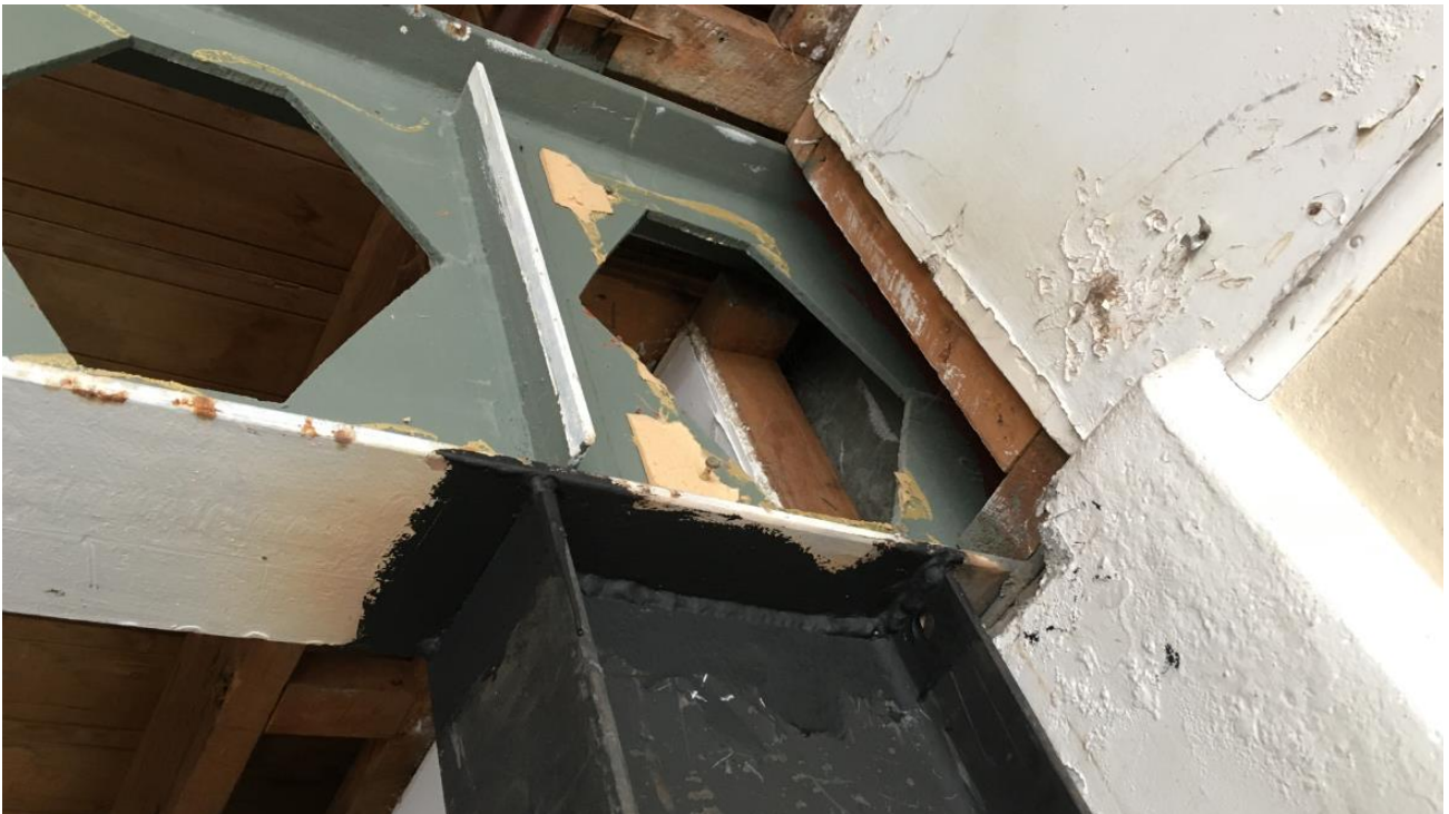
Photo 2 – Column A-2. Top connection
