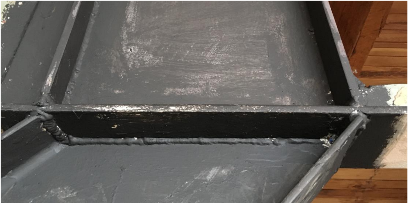
Photo 4 – Column C-2. Top connection
