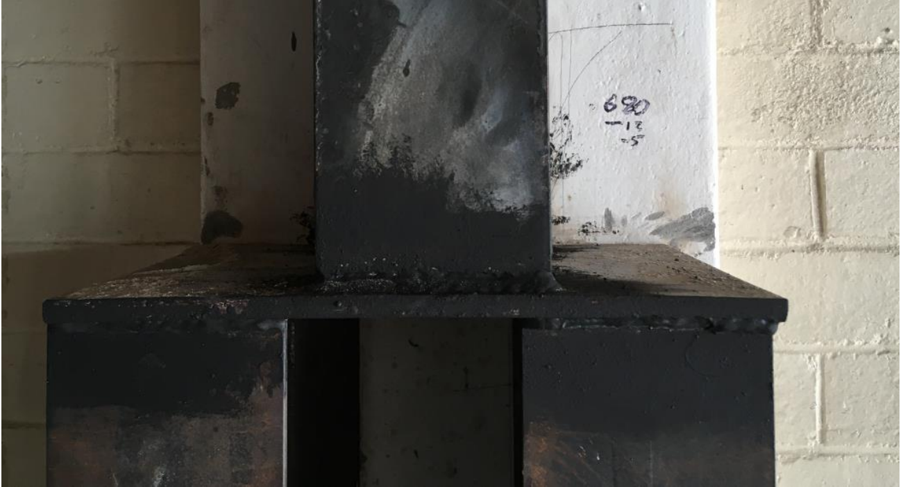
Photo 1 – Column A-2. Bottom connection
