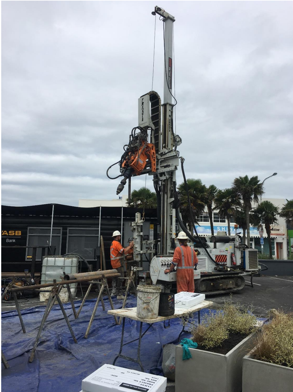
Image 1. Site investigations with sonic drilling rig
