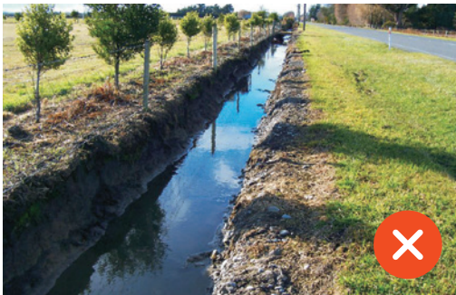
Herbicide spray causing unstable banks
