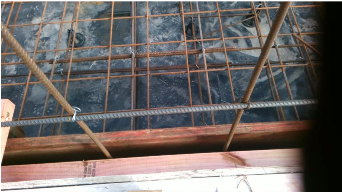
H12 blockwall starters installed @ 400mmc/c Taken at 10:34 AM on Wednesday 22/05/2019 Status: Pass
