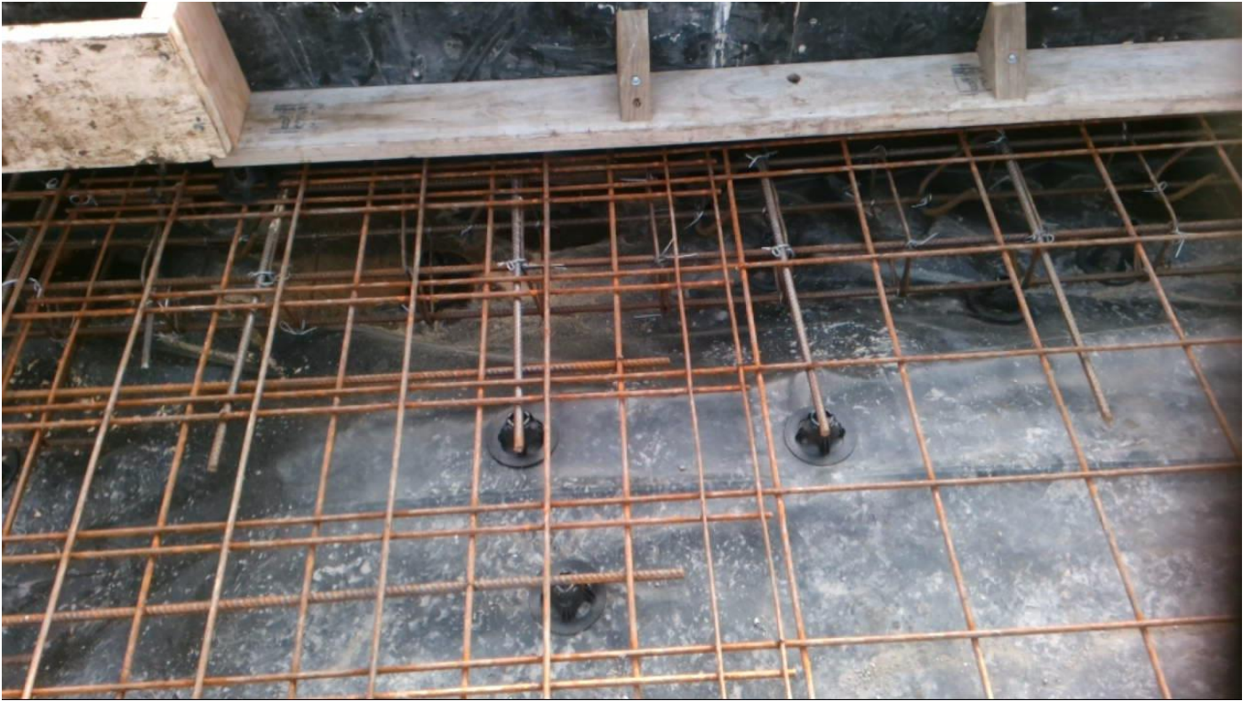
Taken at 10:53 AM on Wednesday 22/05/2019 Status: Pass
