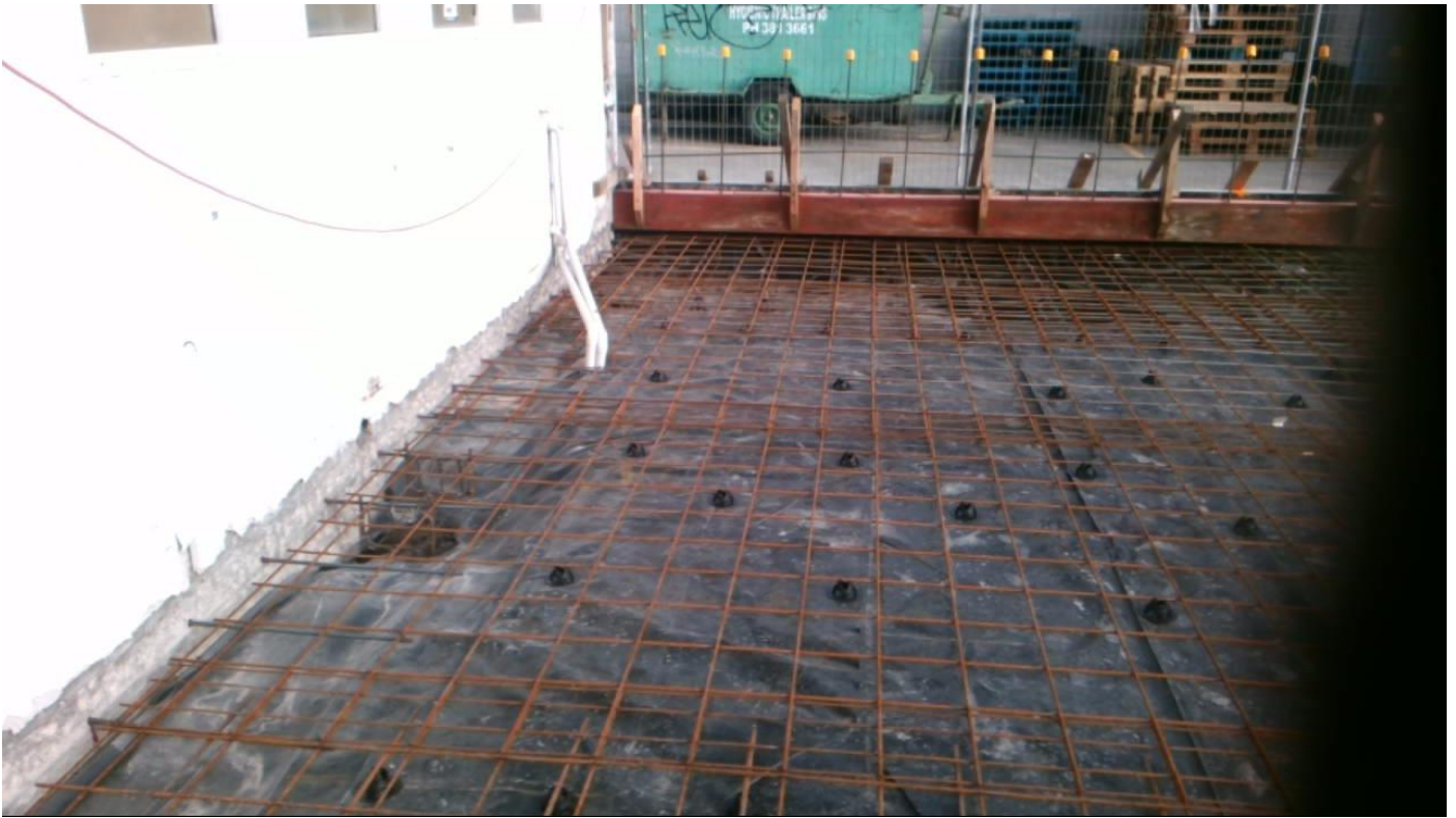
Existing bathroom wastepipes to be made redundant later Taken at 10:32 AM on Wednesday 22/05/2019
