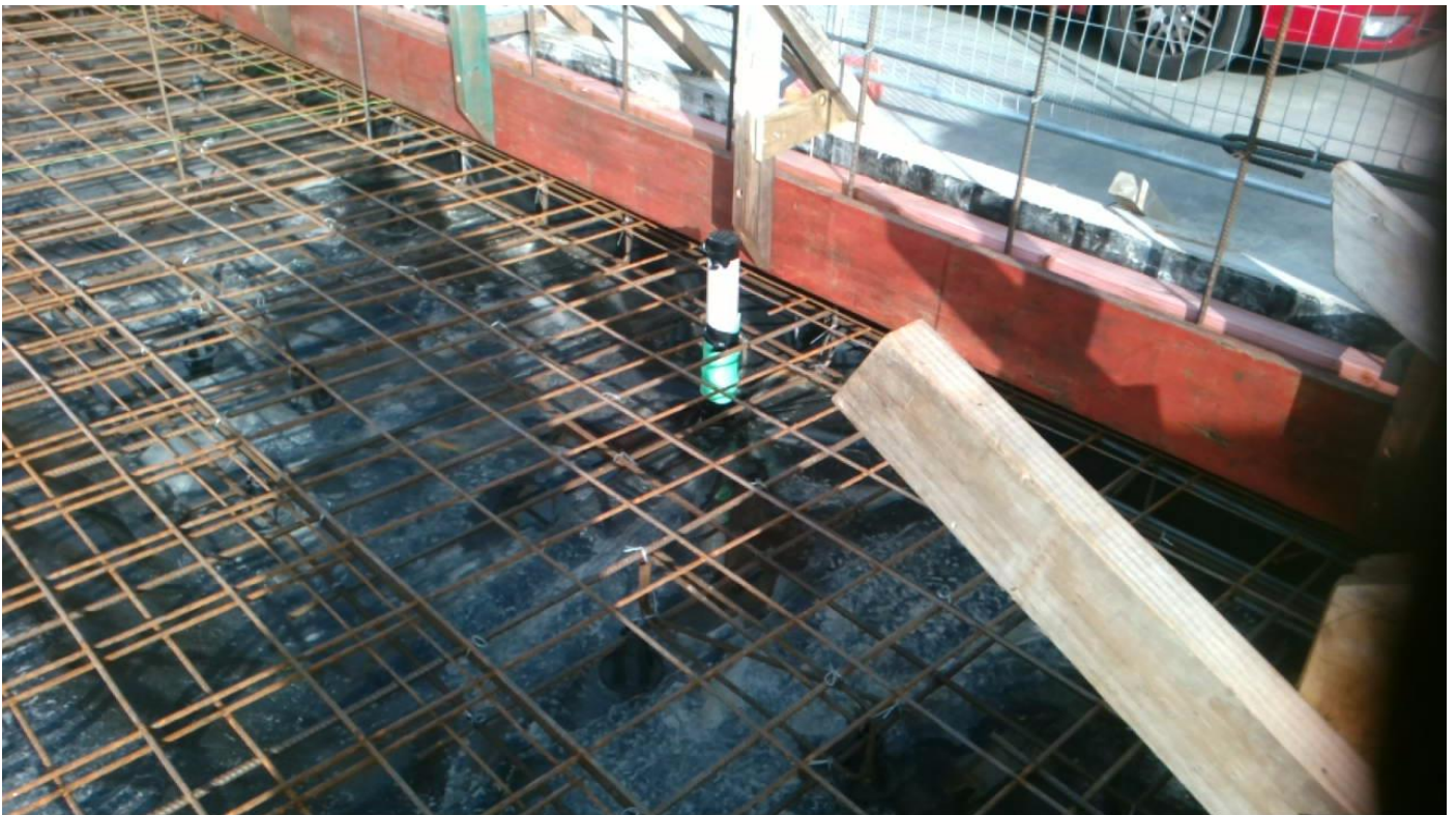
Lagging to be completed higher than concrete Taken at 10:30 AM on Wednesday 22/05/2019
