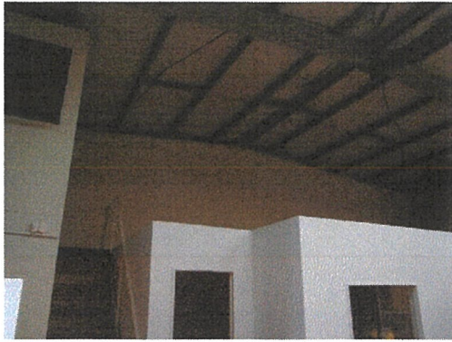
Photo 7 – Rear units with interior offices built on floor
