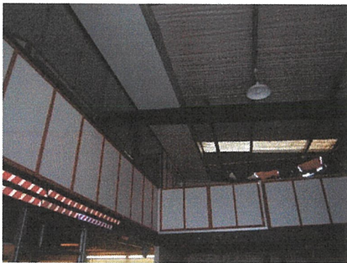
Photo 15 – Unit 1 mezzanine and roof framing
