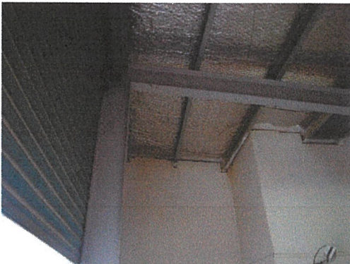
Photo 3 – Front units with drop portal frame at roof
