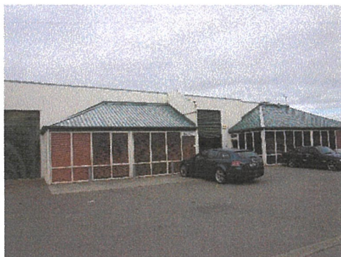
Photo 11 – Offices outside concrete building
