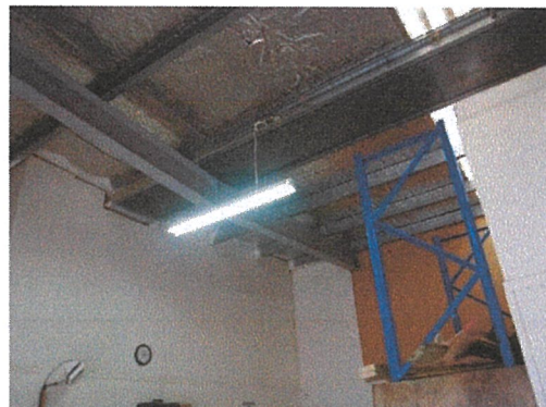
Photo 4 – Front units with drop portal frame at roof with one of two gutters in middle of span
