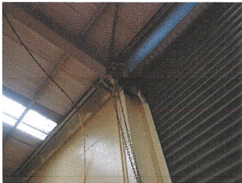
Photo 9 – Rear units with diagonal roof braces and portal knee joint
