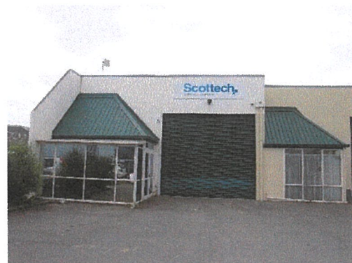
Photo 12 – Offices outside concrete building
