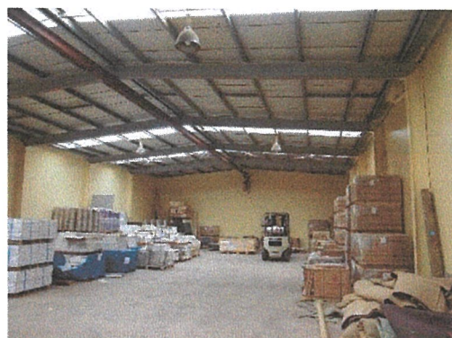
Photo 6 – Interior of warehouse in rear units with ridge portal frames
