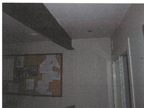
Photo 18 – Roof framing to panel connection
