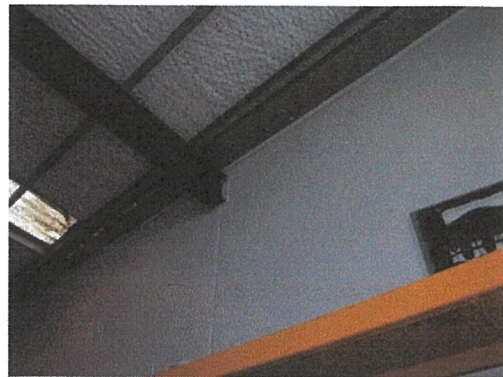
Photo 14 – Portal beam for roof within unit 1
