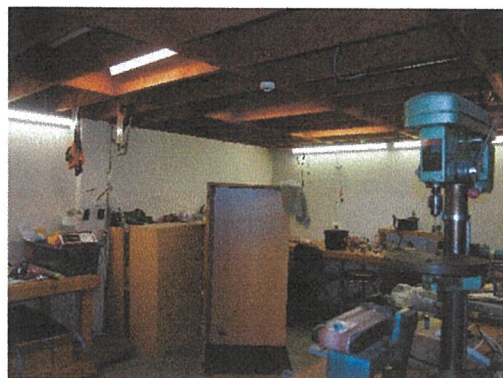
Photo 16 – Underside of mezzanine framing
