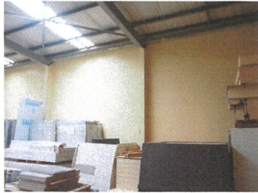
Photo 8 – Rear units with diagonal roof braces and portal
