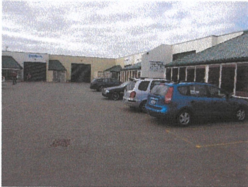
Photo 1 – Street and West South side with front office areas into carpark
