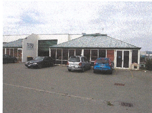
Photo 2 – Front unit at street side
