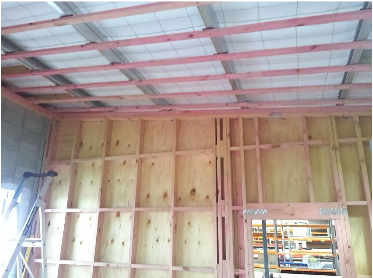
Sample of ceiling battens and wall framing Taken at 1:35 PM on Wednesday 25/09/2019
