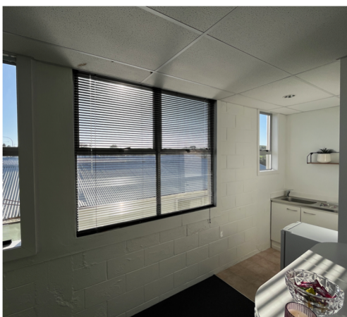
(e) Masonry block on sides of building.
