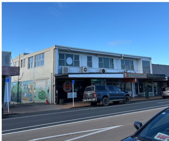
(a) Building Shopfront
