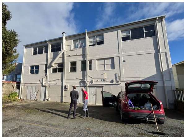
(b) Building Rear
