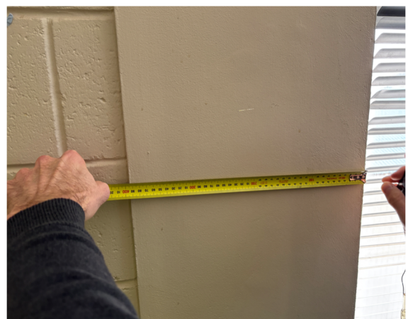
(f) Concrete columns.
