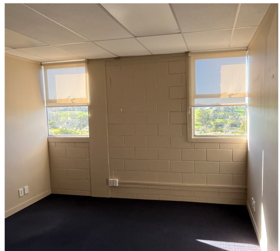
(d) Masonry block on rear of building.
