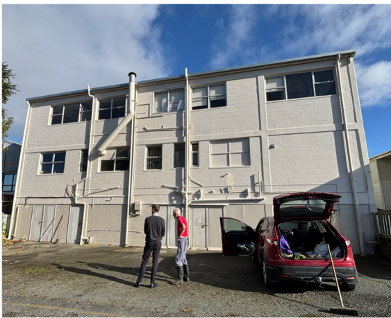
(i) Service areas towards the rear to access the partial basement
