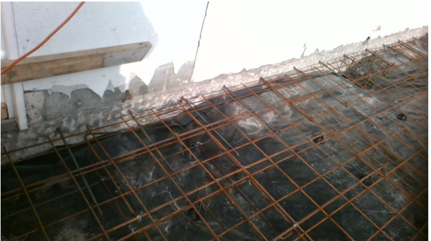
H12 starters epoxied into existing foundations @ 400mmc/c Taken at 10:33 AM on Wednesday 22/05/2019
