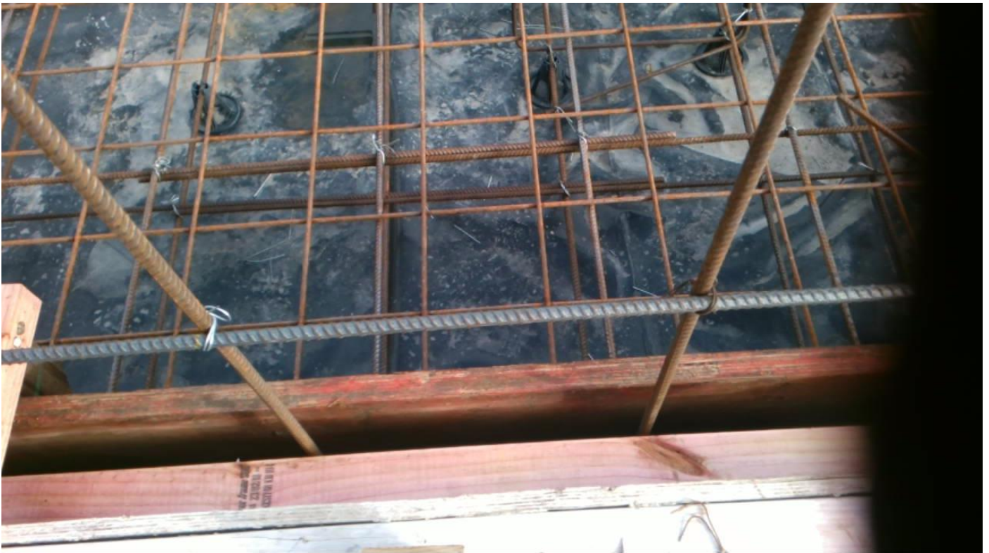
H12 blockwall starters installed @ 400mmc/c Taken at 10:34 AM on Wednesday 22/05/2019 Status: Pass
