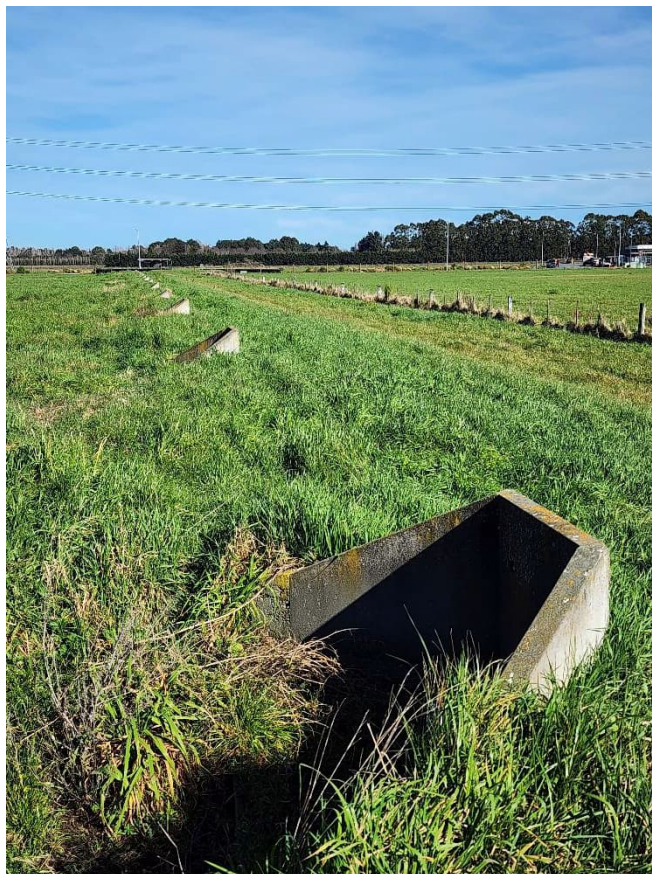
Photograph 9: Southern headstocks Block 2 looking west. (August 2025 Investigation).
