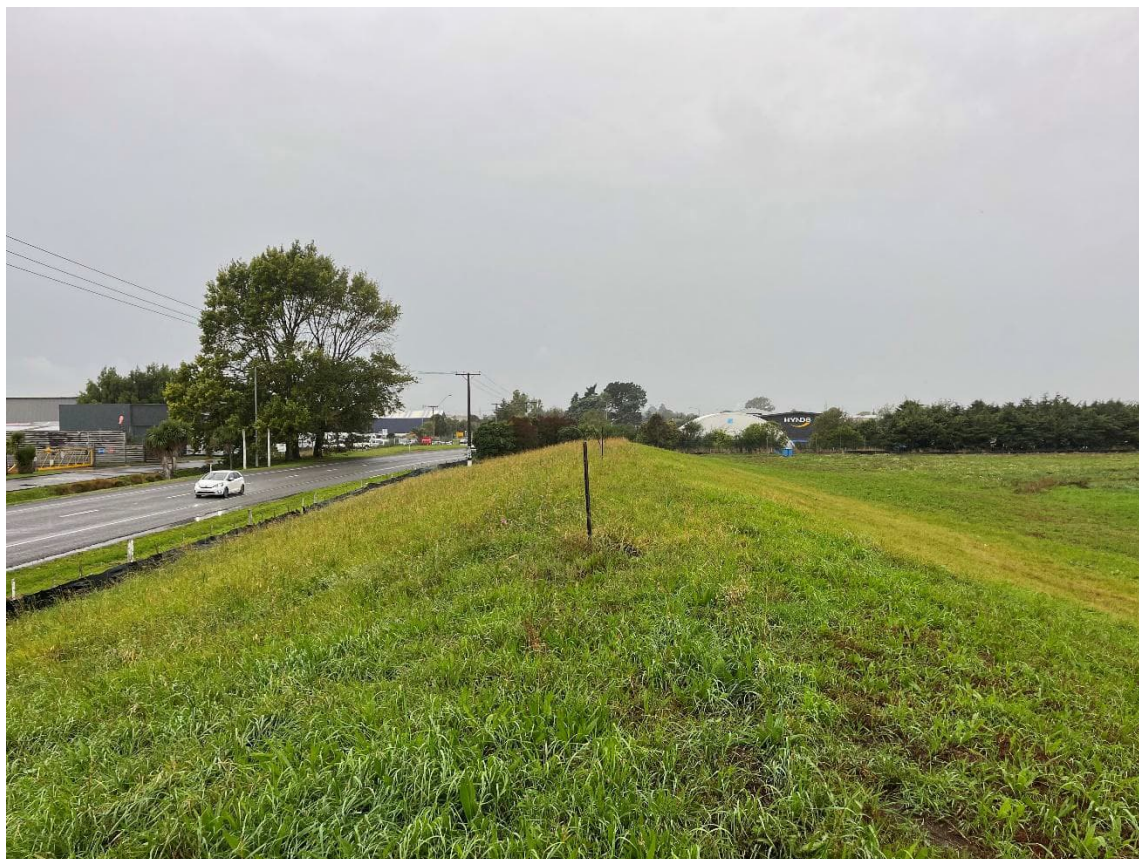
Photograph 8: View of the encapsulated bund looking east. (March/April 2025 Investigation)
