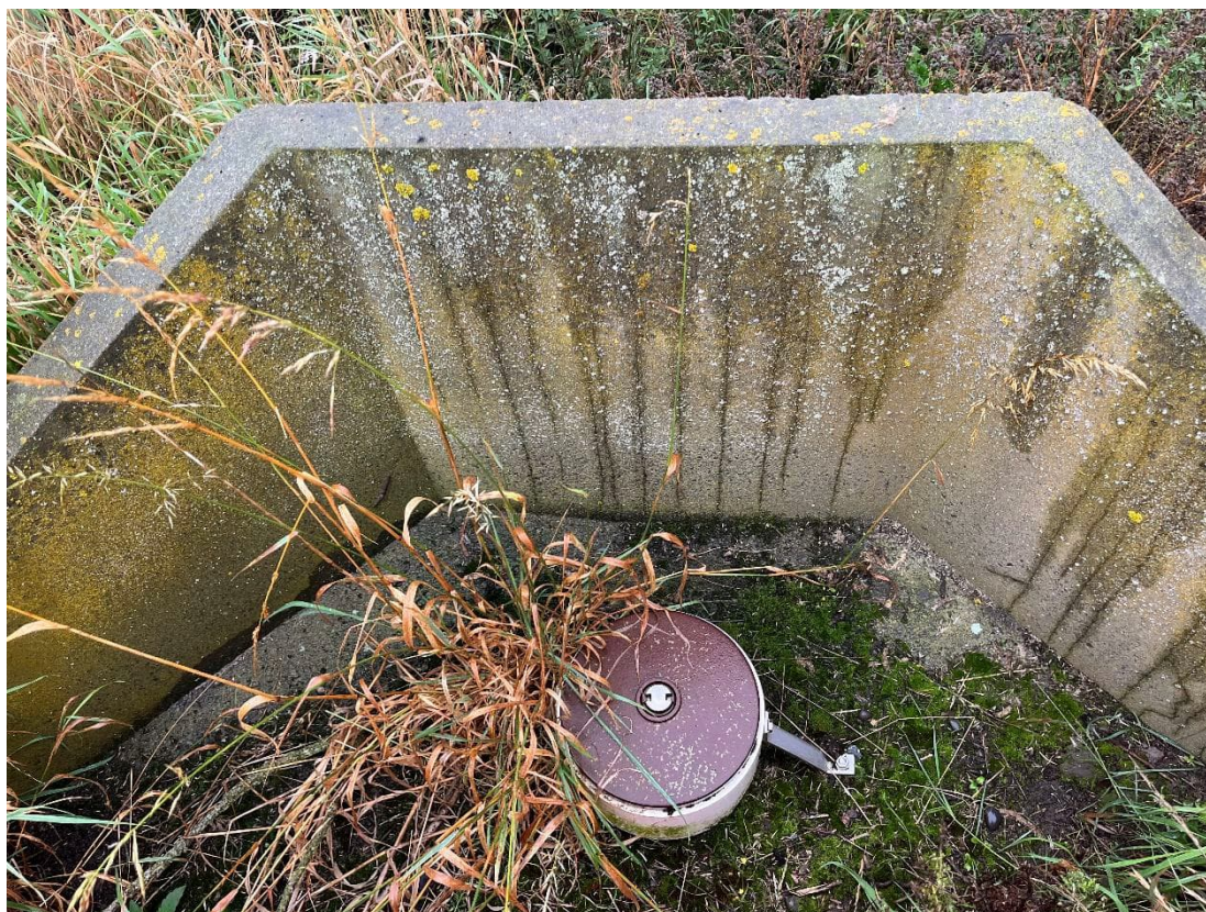
Photograph 4: A remaining headstock in Block 1. (March/April 2025 Investigation).
