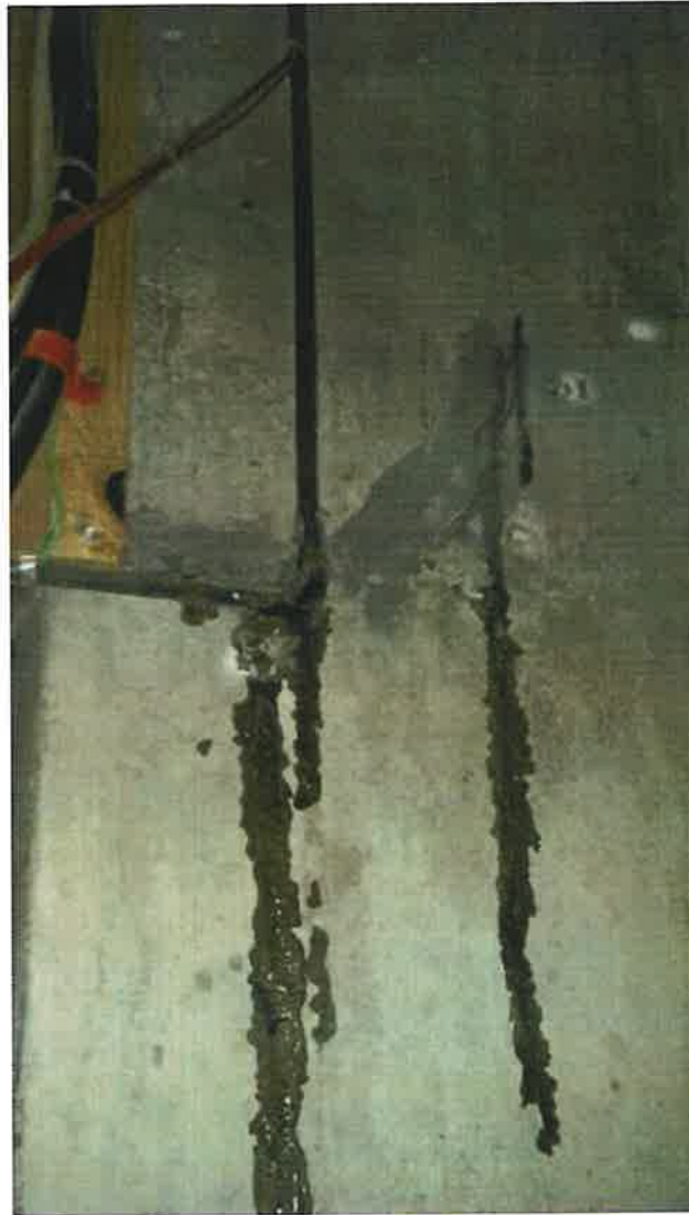
EQ repairs carried out
