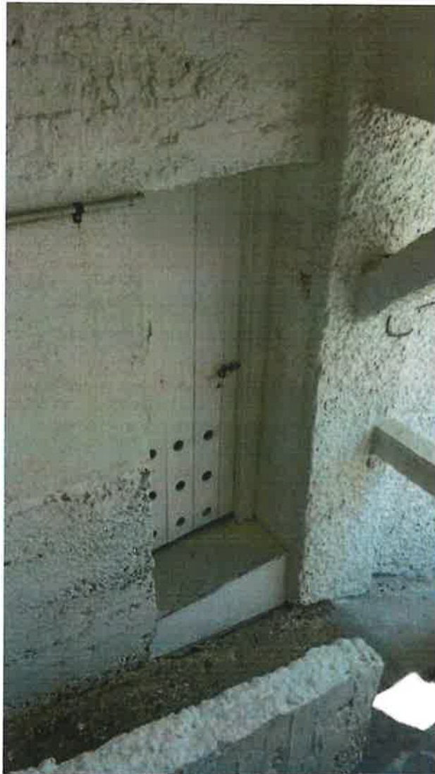
Trap door to subfloor repairs
