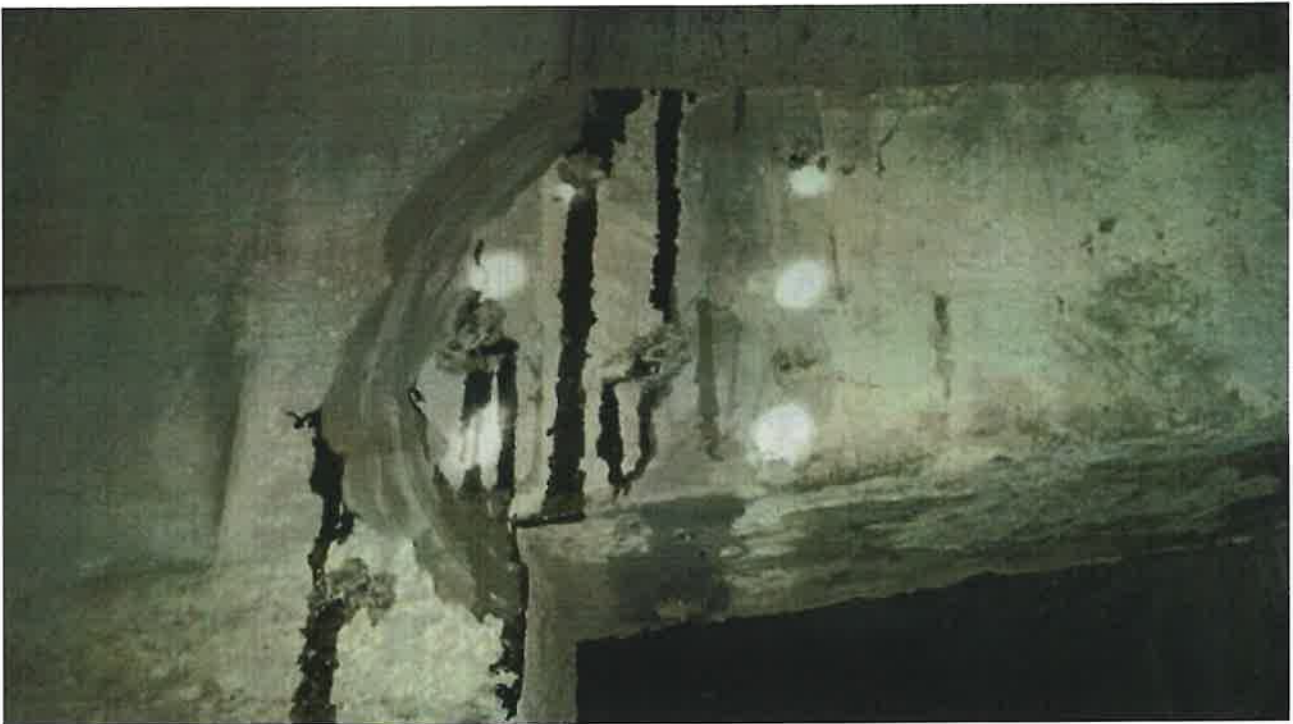
EQ repairs carried out
