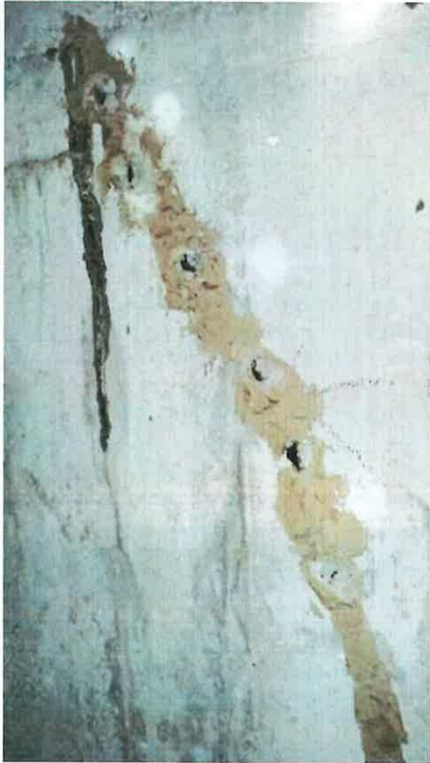
EQ repairs carried out
