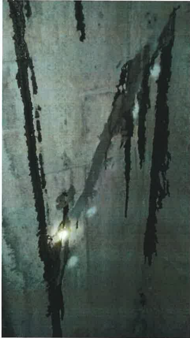
EQ repairs carried out
