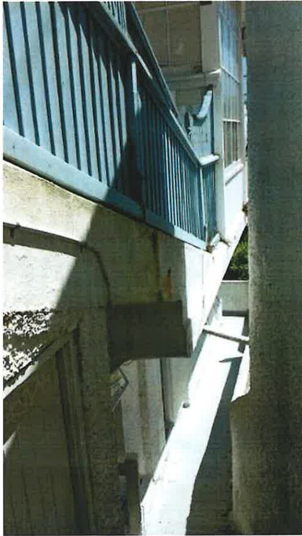
Side elevation of flat B and where concrete fractures were repaired
