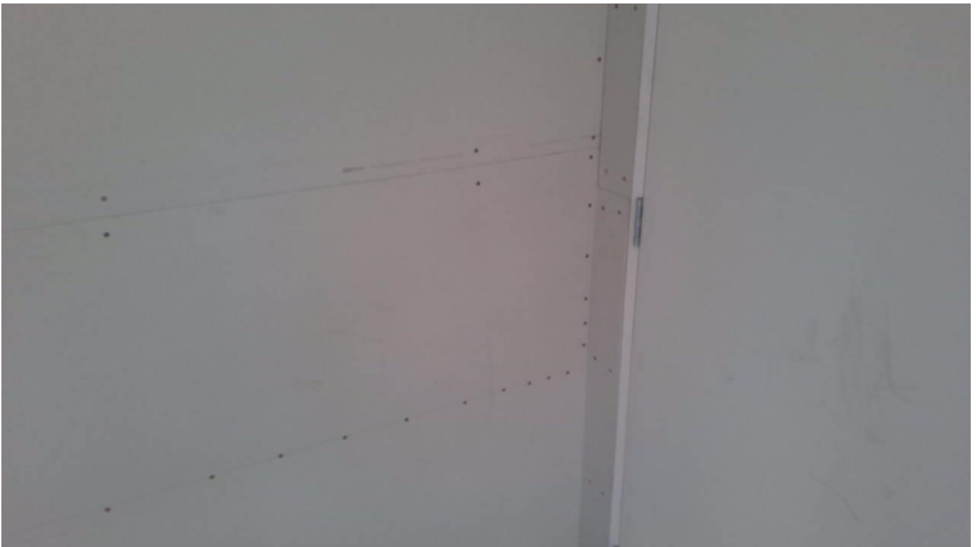
corner of brace unit Taken at 12:04 PM on Tuesday 26/11/2019
