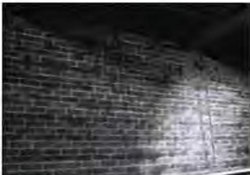
Figure 3 Close up of interior brick wall
