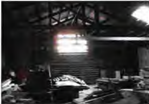
Figure 6. Interior view showing east end timber framed wall
