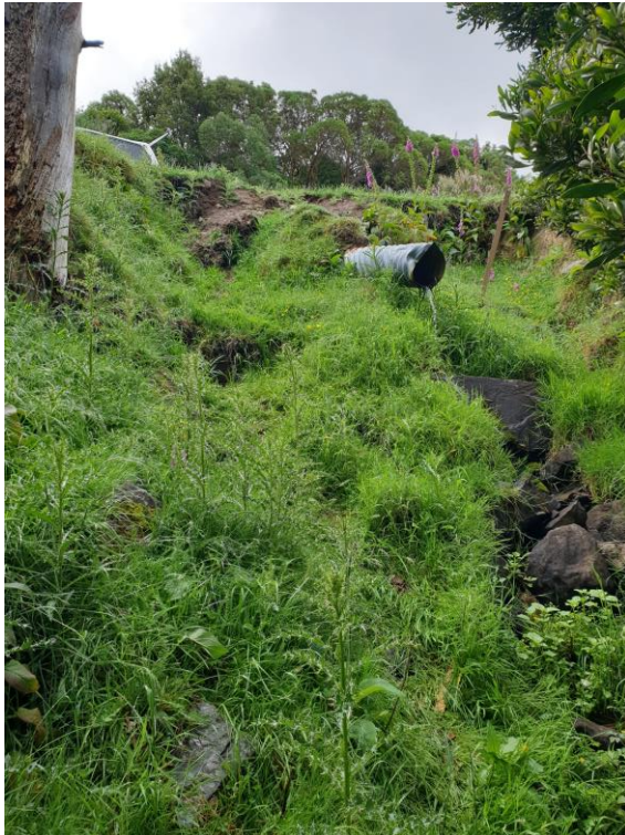
Image 2 - Image showing slope below culvert outlet where MSE wall will be constructed.
