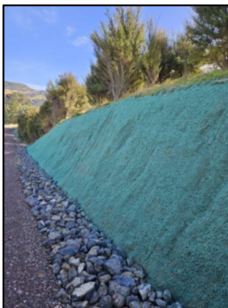
Figure 1: Figure provided by Survus showing accessway slope stabilisation works.
