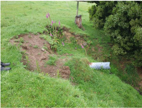
Image 1 - Image showing scoured soil above culvert outlet.
