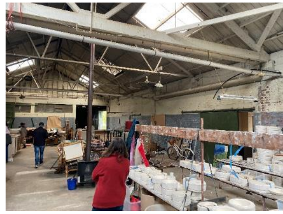
Photo 22 – Building 4B Interior
