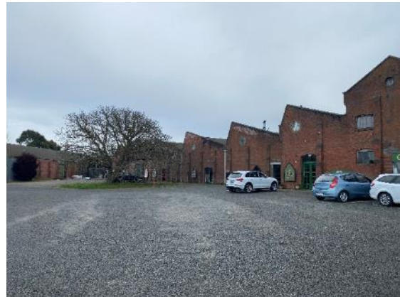
Photo 2 – Site Front Elevation
