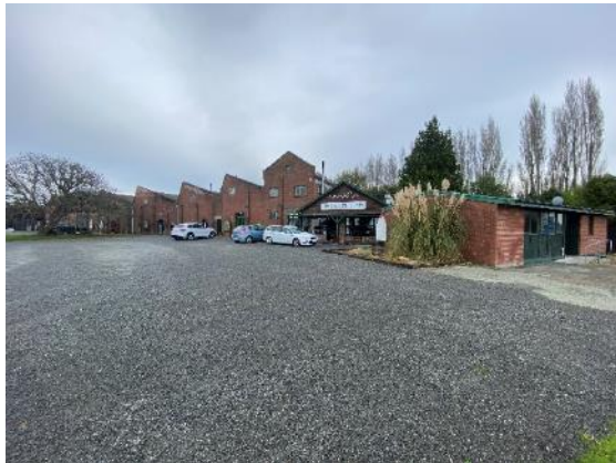
Photo 1 – Site Front Elevation
