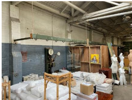
Photo 21 – Building 4B Interior
