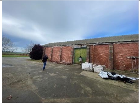
Photo 26 – Storage Building Exterior
