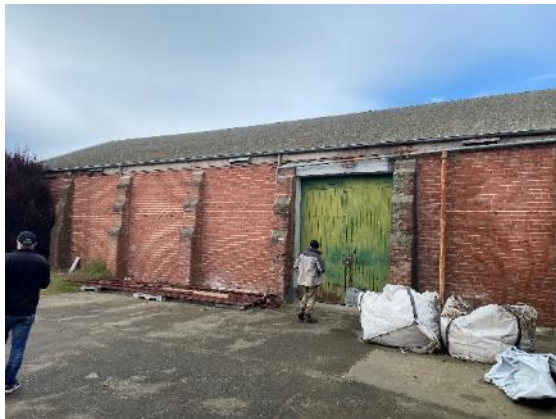
Photo 27 – Storage Building Exterior
