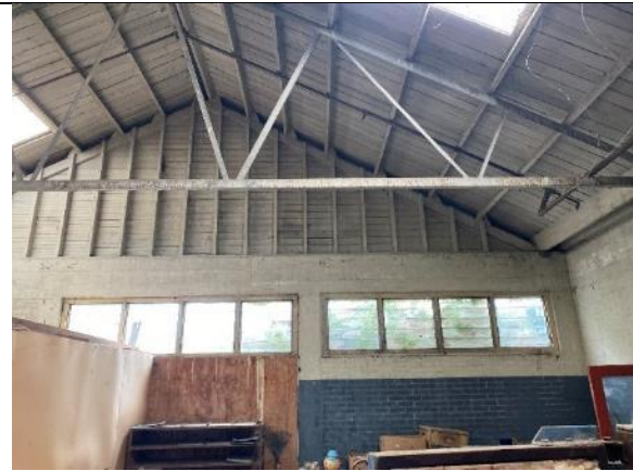
Photo 20 – Building 4A Interior
