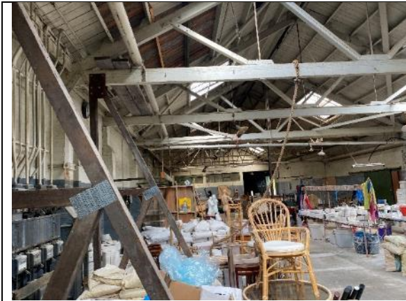
Photo 19 – Building 4A Interior
