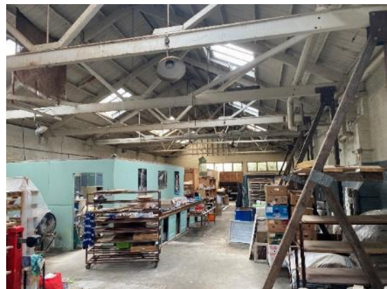
Photo 18 – Building 4A Interior
