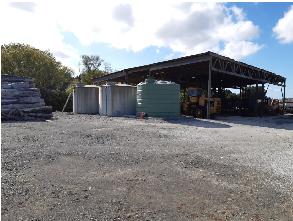
Figure 5. View east towards the water tanks and where trucks will fill up.
