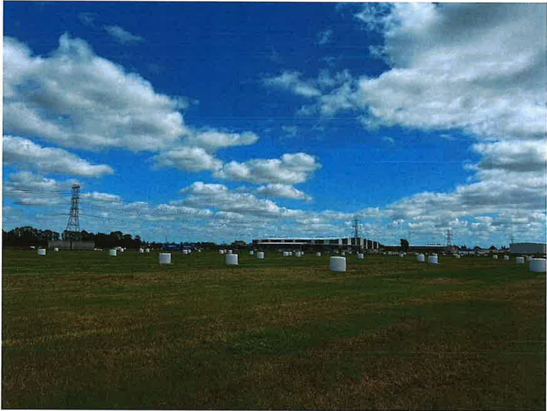
Photograph 1: View of Block 2 looking north-west (March/April 2025 Investigation).
