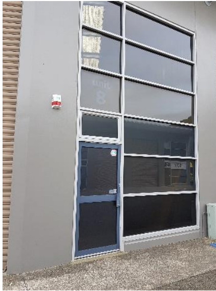
Figure 18: Windows from Central Block appears to be in good condition.
