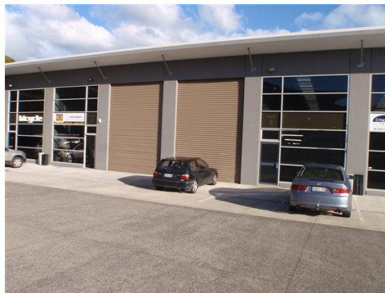
Figure 14: Carpark lines between Southern and Central Block appear to be satisfactory
