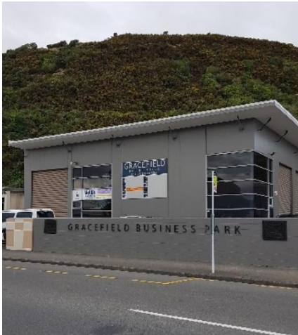
Figure 17: The Central block recently painted in excellent condition.
