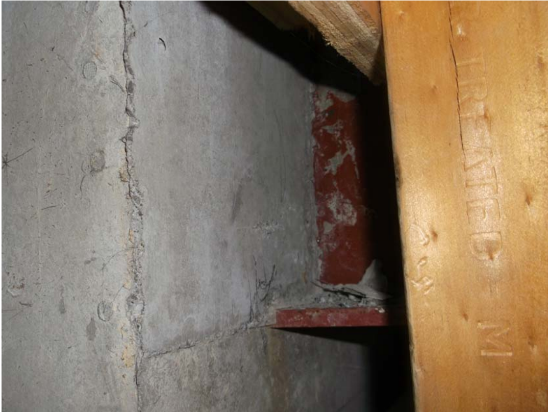
Figure 5 - Roof beam to first floor column connection
