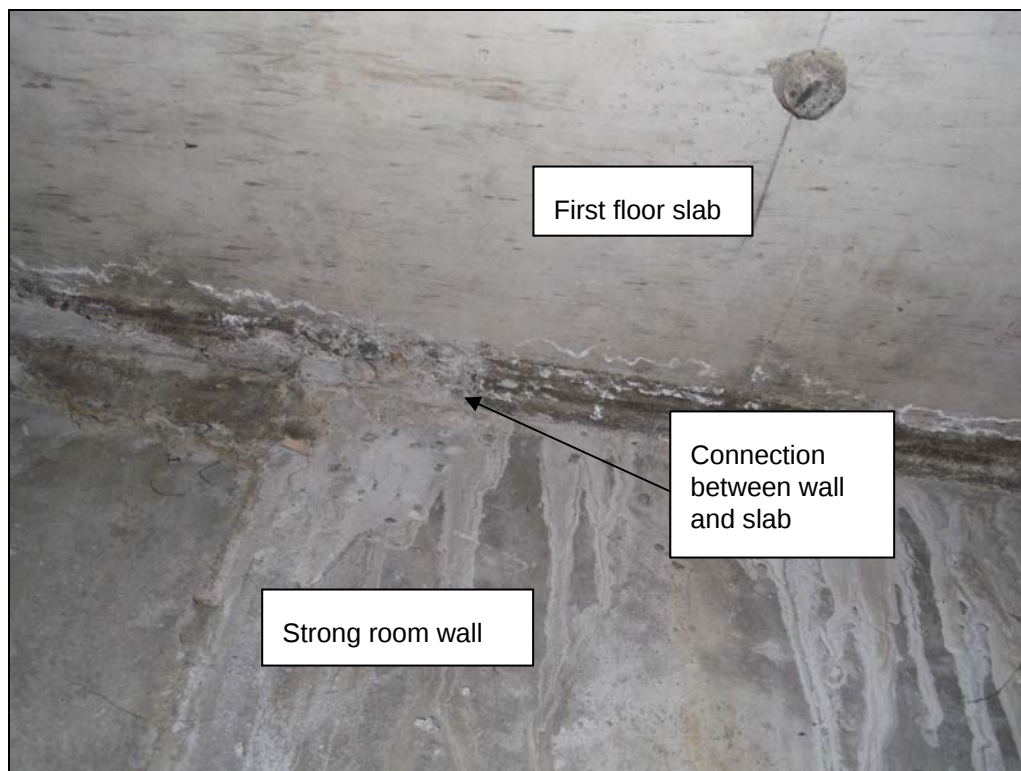
Figure 4 - Strong room to first floor slab connection
