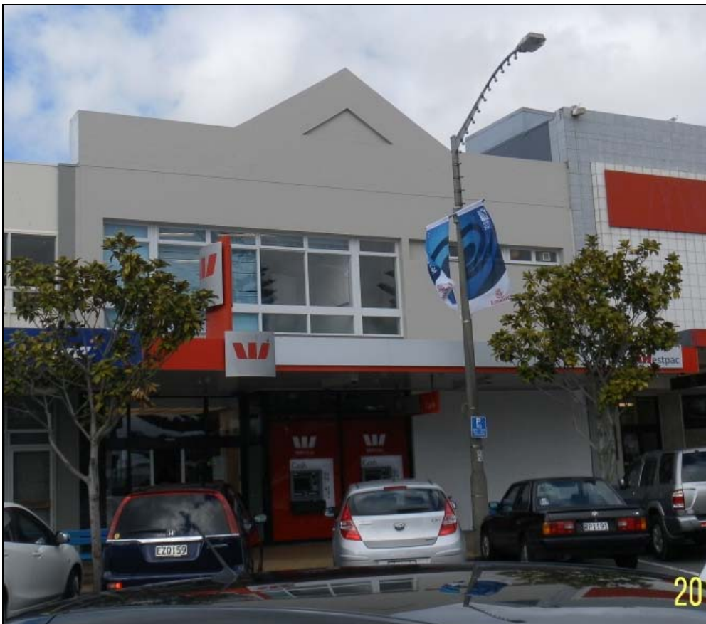
Figure 2 – Porirua Branch, 2 Cobham Court
