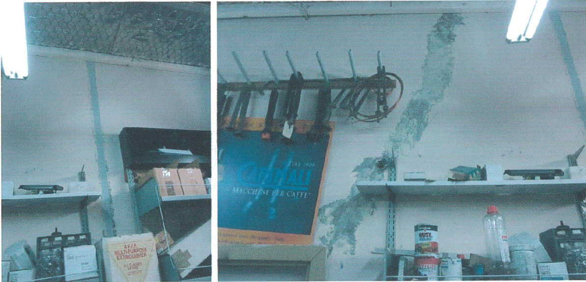
Unit 7 additional wall repairs.
