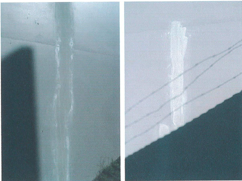
Unit 9 additional wall repairs.
