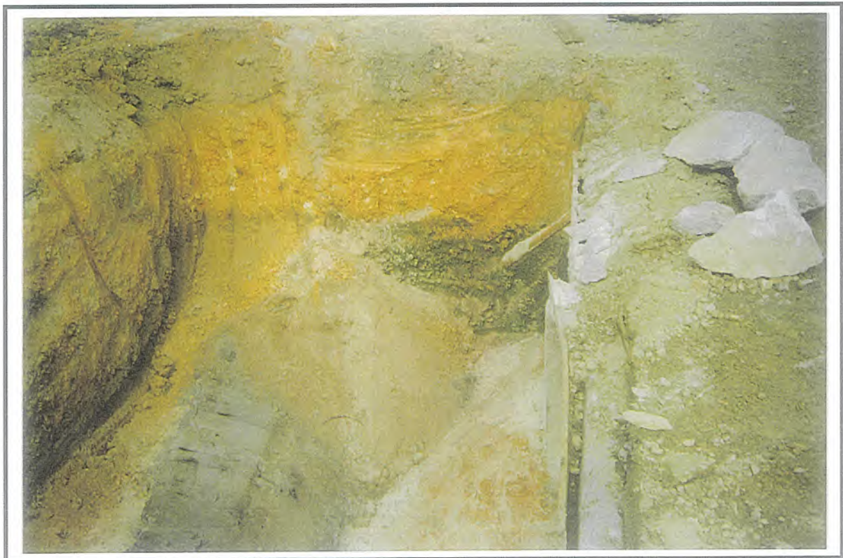
Photo 4: The tank-pit after removal of the first tank, showing the base material that was subsequently removed.
