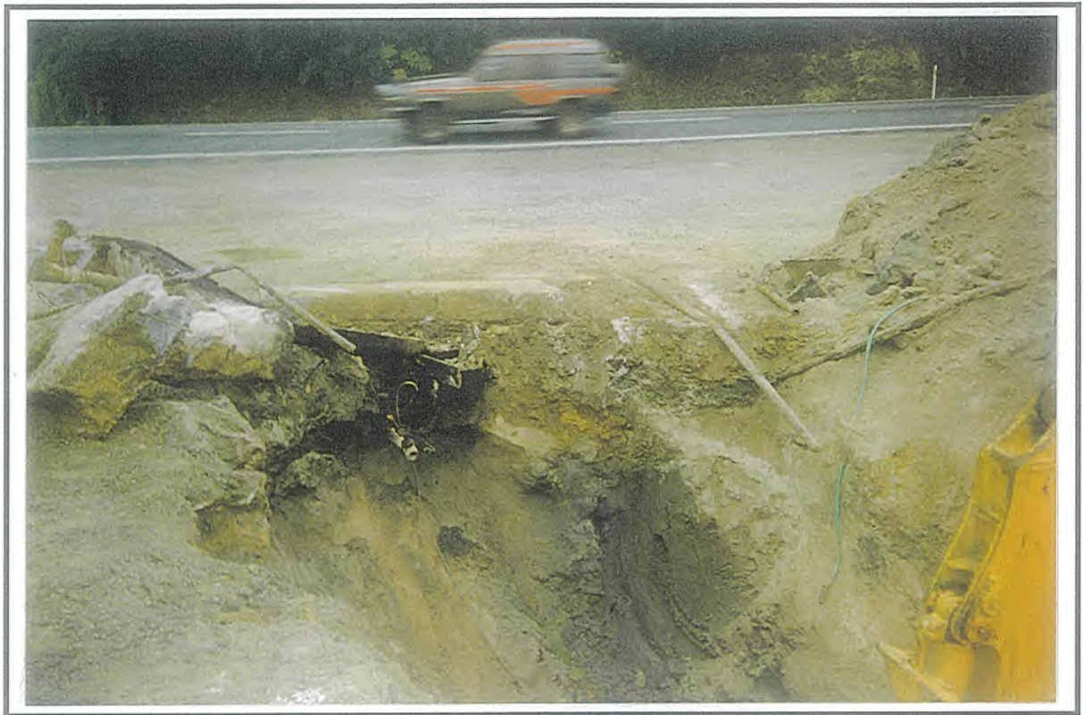
Photo 5: The tank-pit after removal of the second diesel tank. The pumps were located at the end of the pit, and the dark soils beneath them were removed.
