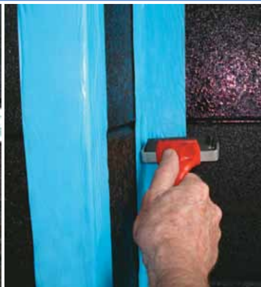
B – Gussets installed in high stress areas
