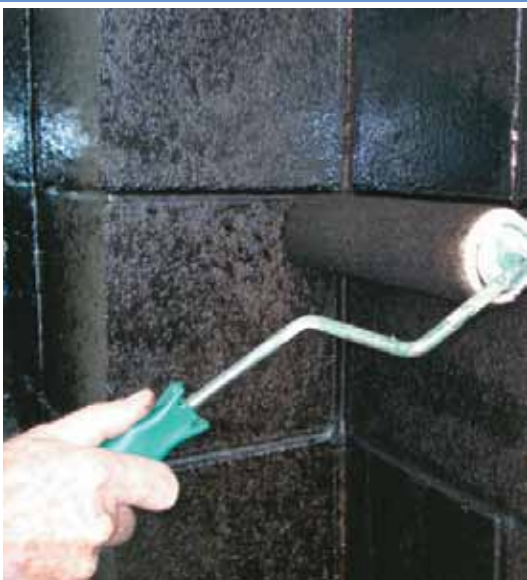
A – Nuraflux primer applied to substrate
