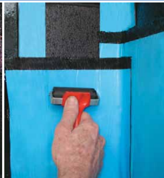
C – Roller used to ensure good seal
