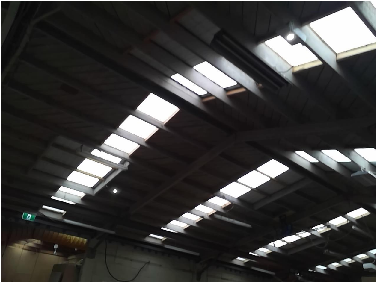
Exit sign + emergency lighting Taken at 8:41 AM on Friday 7/02/2020
