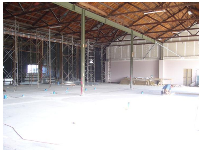
Photo 13: Existing Construction Photos (Dated 2009)
