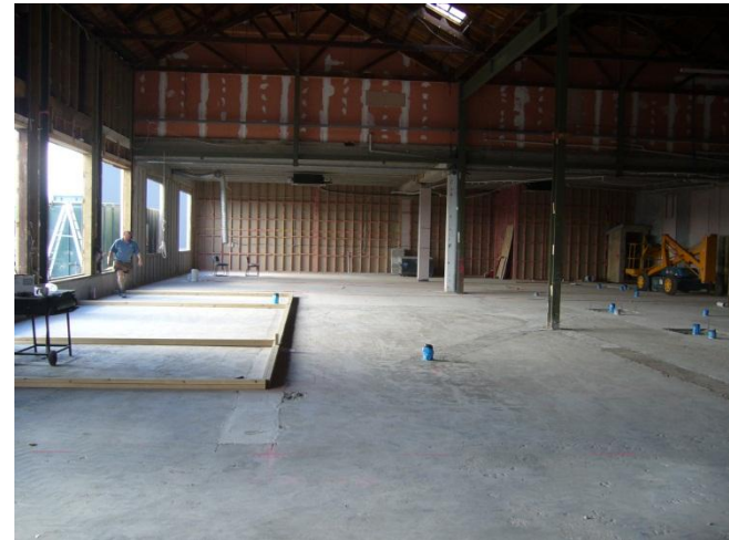
Photo 12: Existing Construction Photos (Dated 2009) of Part 3
