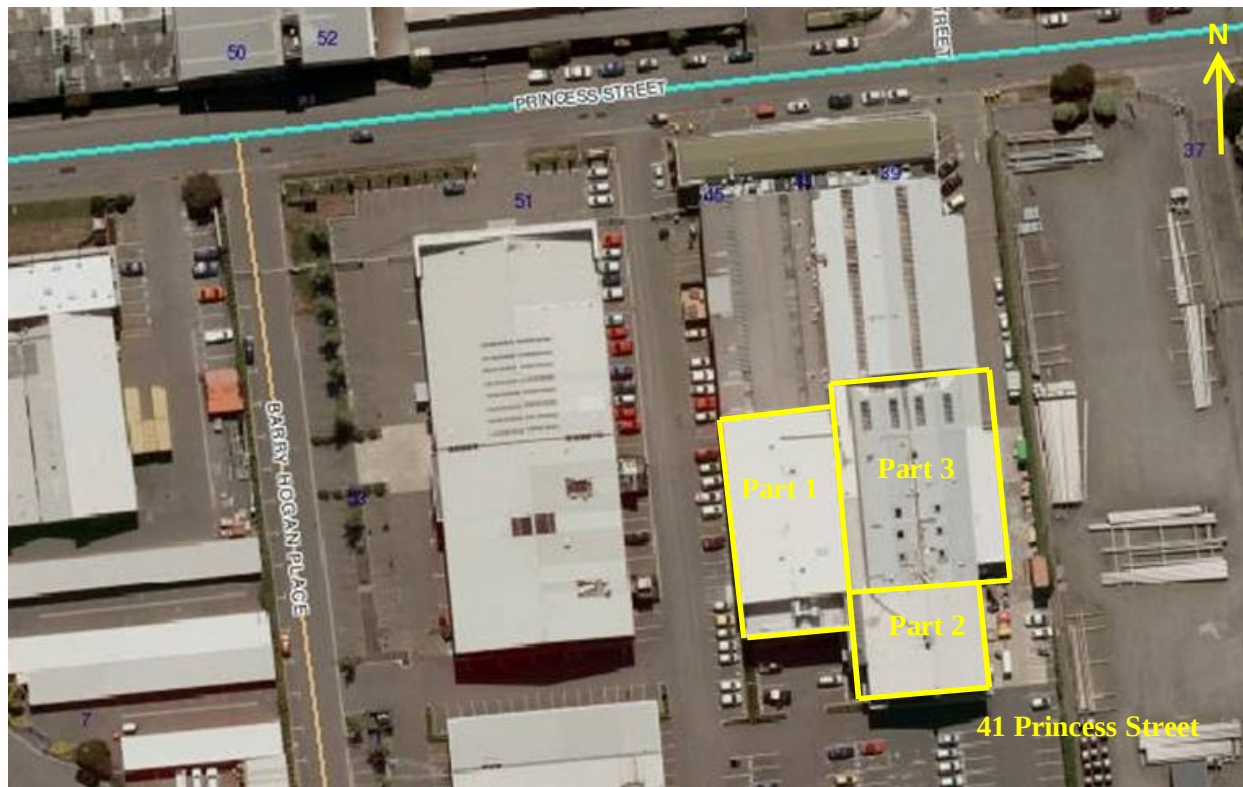
■ Figure 1 Aerial Photograph of 41 Princess Street
