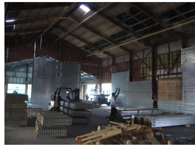
Photo 14: Existing Construction Photos (Dated 2009) of Part 3
