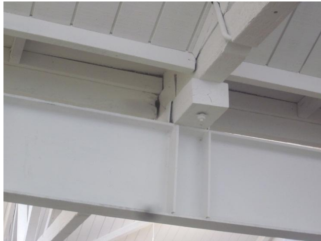
Photo 11: Part 3 – Roof Truss Connection to Spine Beam
