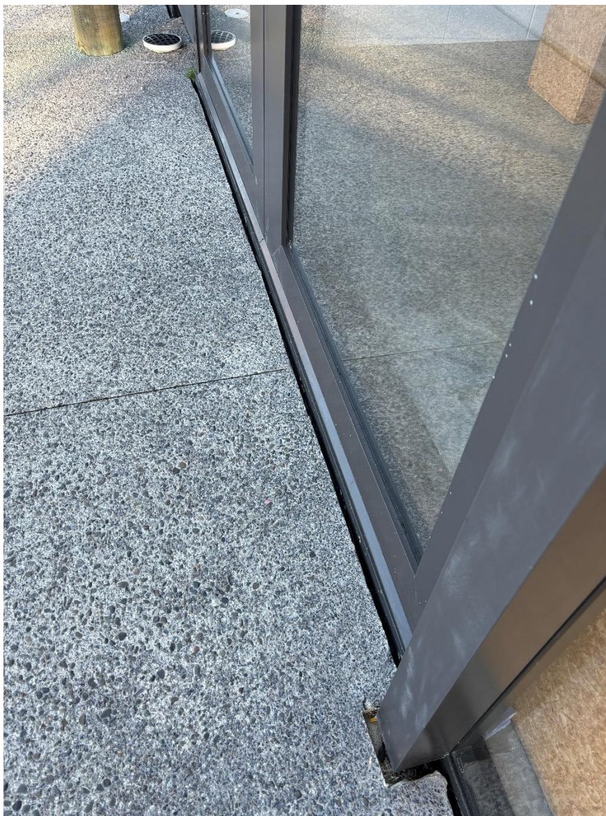
“Construction Gap” - cleared and clean
