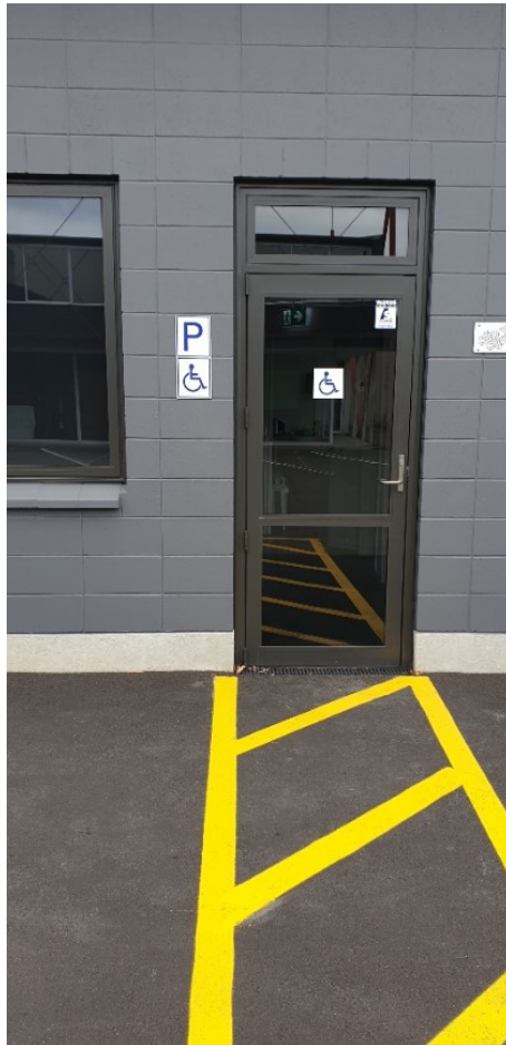
ISA sign installed
