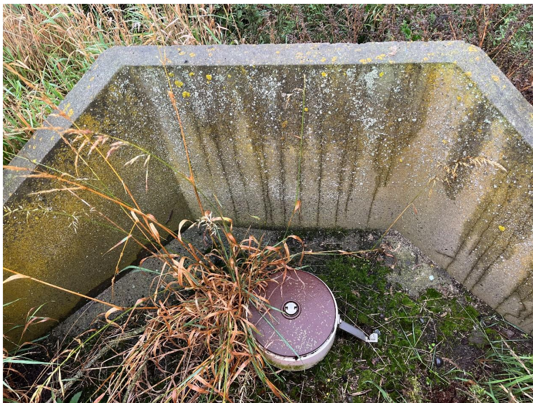
Photograph 4: A remaining headstock in Block 1. (March/April 2025 Investigation).
