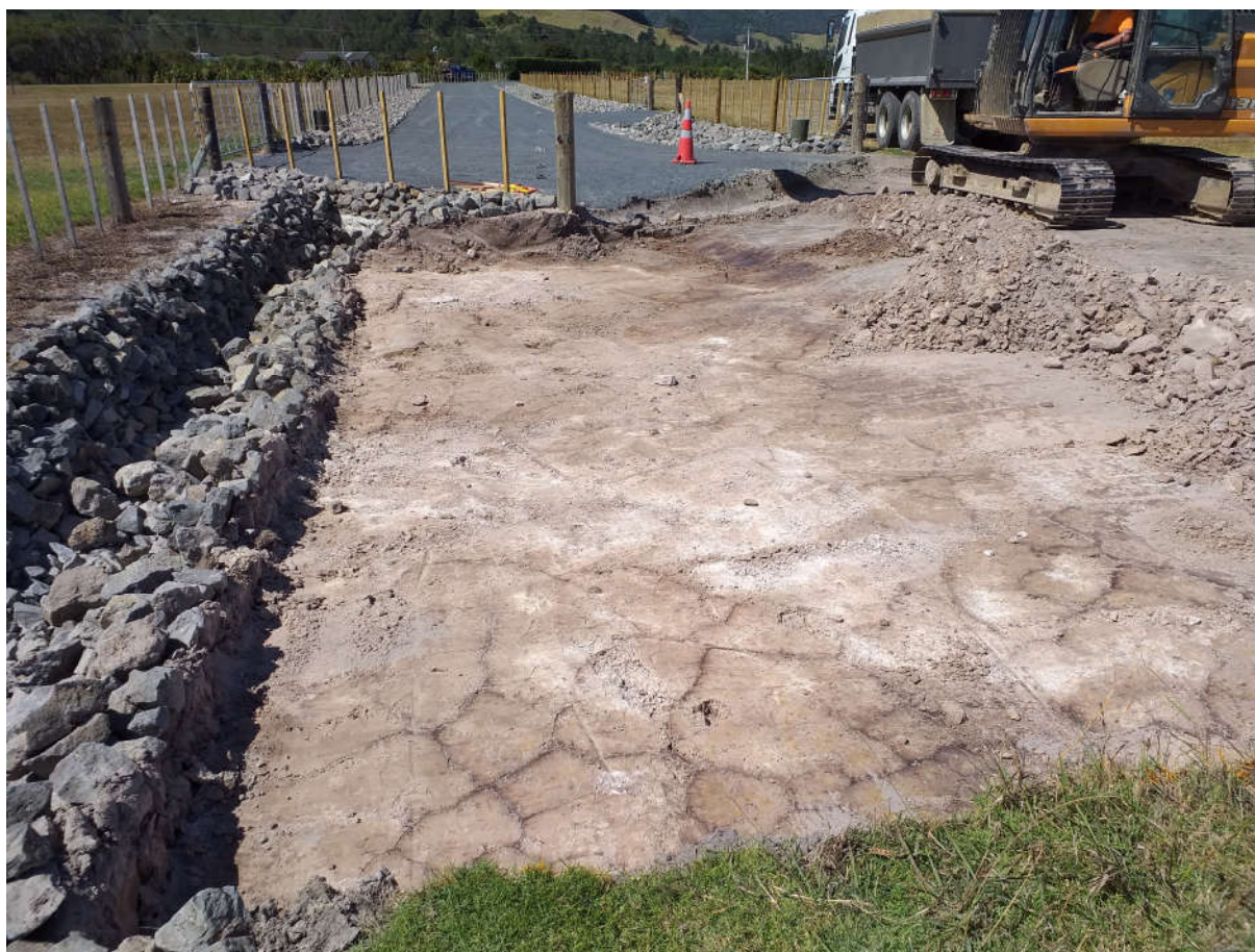
Figure 3 – Evidence of soil desiccation below ground surface and hard pan layer
