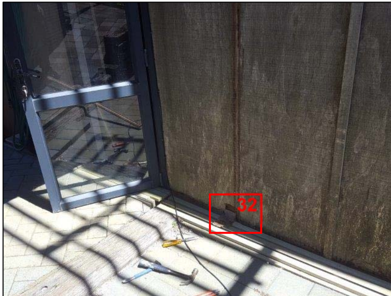
Photo 31: Cladding cutout at bottom plate on garage NE elevation. Refer photo 26 for location and next photo for cutout
