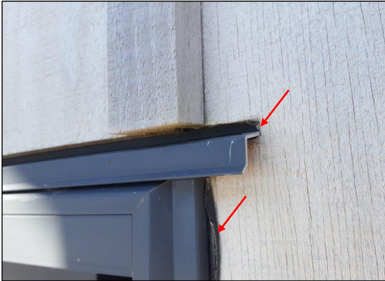
Photo 67: Cladding junction at end of master bedroom head flashing appears to be reasonably well installed (other end similar). Inseal strip is visible behind the jamb flange
