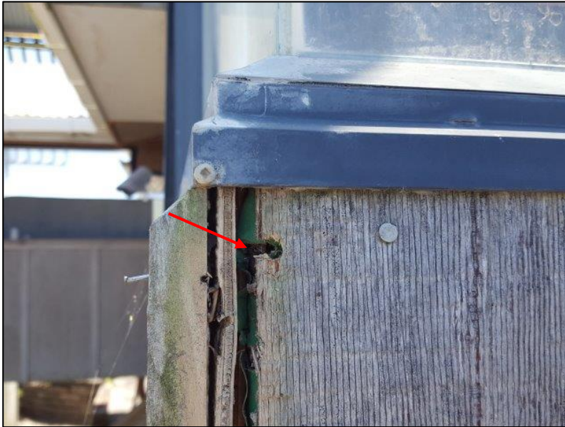
Photo 13: Bathroom external corner. The cover batten was loose and there are gaps in the building paper (indicated). The gap between the cladding sheets is larger than the 2-3mm expansion gap required by the manufacturer. No corrosion issues were noted with the cladding fixings. Refer next photo
