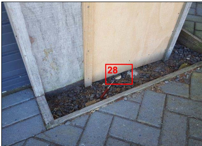
Photo 27: Plywood cladding has been replaced on SE garage elevation. Refer Dodd drawings (Minor Alterations 2). Ground clearances don't comply with drawings or meet Acceptable Solution. Refer Appendix C for photograph of bottom plate framing taken by builder. It appears the condition of the timber wasn't independently verified by the building surveyor
