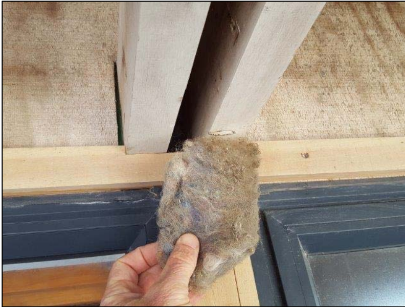
Photo 88: Piece of insulation only in large gap between timber truss bottom chords
