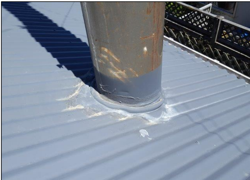
Photo 96: No issues were noted with the roof structure. The curved long run profiled steel roofing appears to be well installed, including the pictured chimney junction
