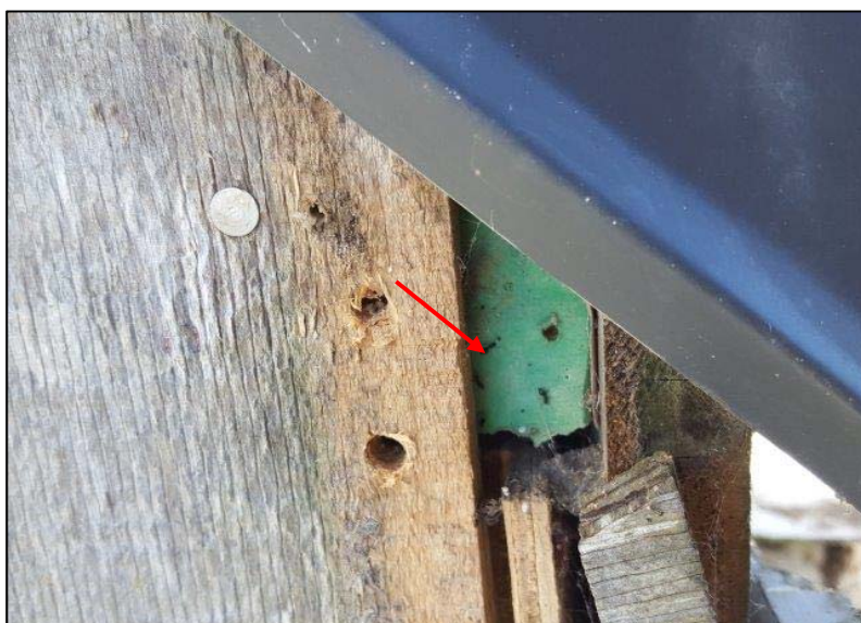
Photo 18: Lots of ants present at workshop external corner. No galvanised steel flashing was installed. Refer following photos for investigation at bottom plate level
