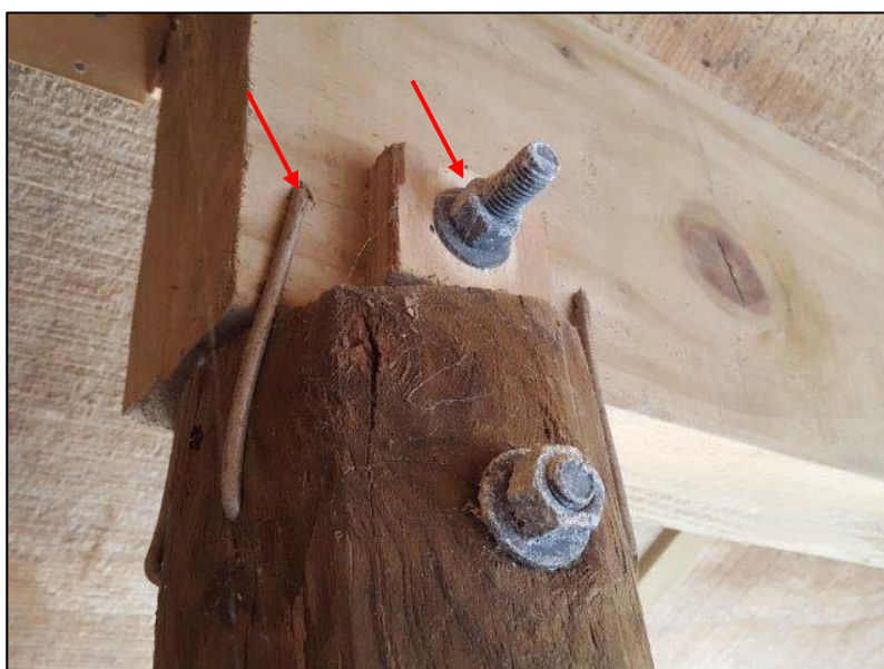
Photo 93: Top beam connection to timber pole is reliant on a single bolted connection and four wire dogs, all in the lower third and close to the end of the beam. The connection is required to perform for the life of the building (i.e. minimum 50 years). The adequacy of the connection is questionable in a major seismic or storm event
