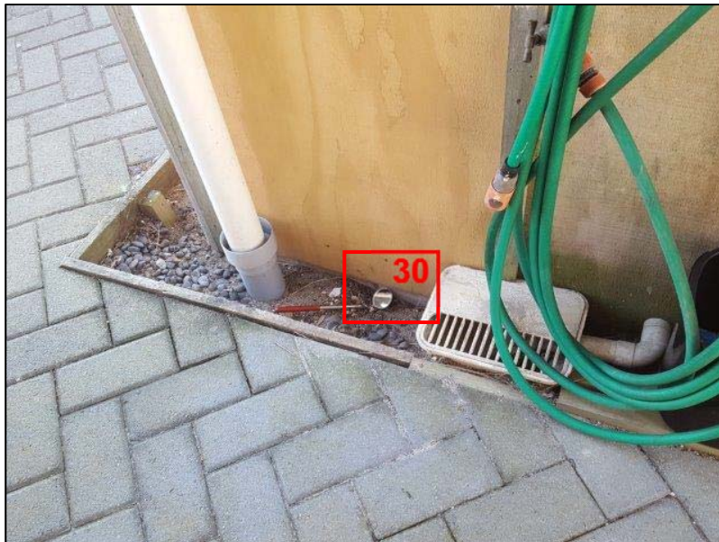
Photo 29: Plywood cladding has been replaced on NE garage elevation. Refer Dodd drawings (Minor Alterations 2). No independent verification provided of timber condition. Refer next photo
