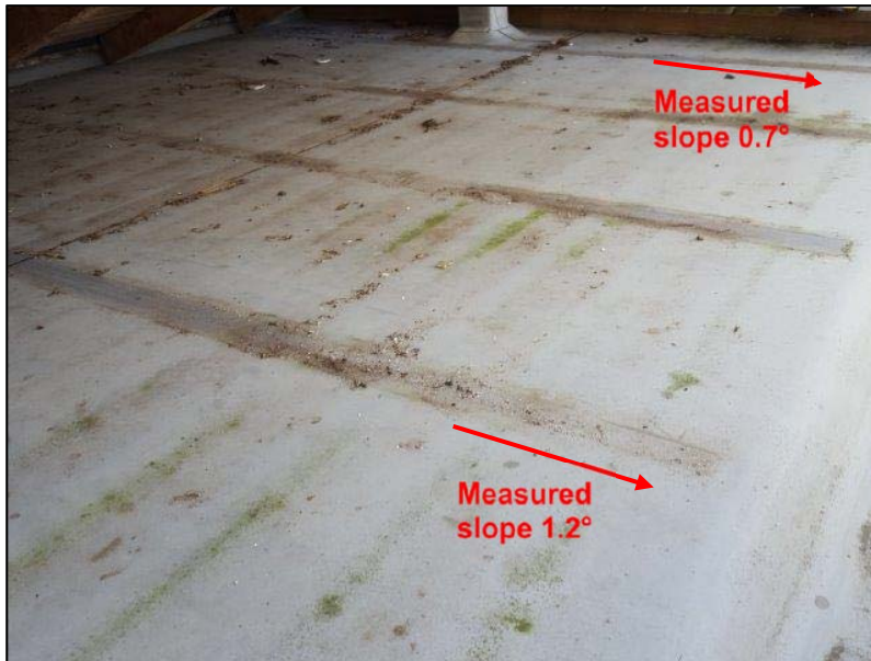
Photo 49: Butyl rubber deck cladding appears to be reasonably well detailed below central section of floating decking. Deck slope was minimal, measured at 1.2° and 0.7° in two locations. No evidence of failure was noted in the garage below and the butyl rubber membrane is protected by the decking
