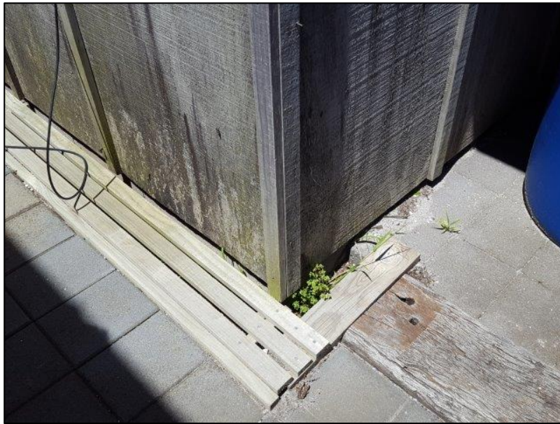
Photo 34: Minimal ground clearance at north corner of garage. Refer Dodd drawings for planned remediation (Minor Alterations 2).
