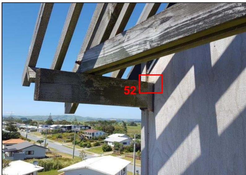
Photo 51: Typical beam penetration through gable cladding. Refer closeup of junction in next photo
