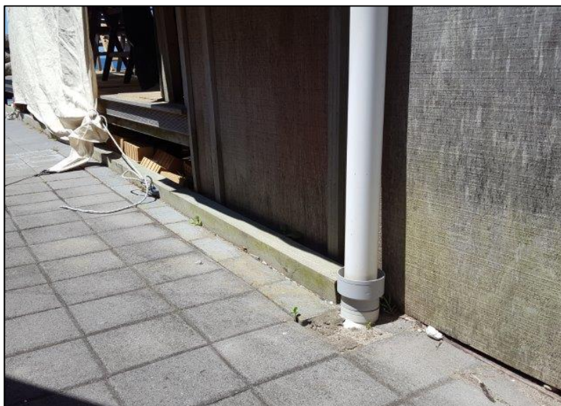
Photo 36: Minimal ground clearances on rear NW house elevation. Refer Dodd drawings for planned remediation (Minor Alterations 2)
