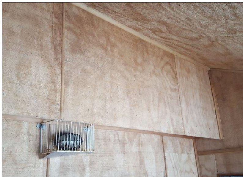
Photo 81: Plywood cladding in house entry area on SW elevation. Cladding has been neatly finished, with trims installed at plywood junctions
