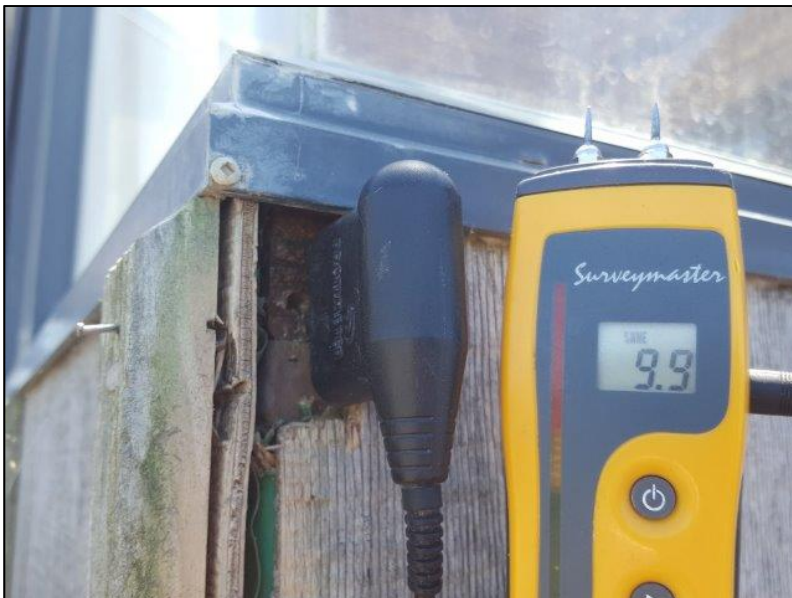
Photo 14: Cladding cutout at external corner. No galvanised steel flashing was installed over the building wrap (recommended by BRANZ). Framing was dark and ants were present (indicating nearby moisture source), MC 9% normal moisture reading taken. Refer next photo for interior view
