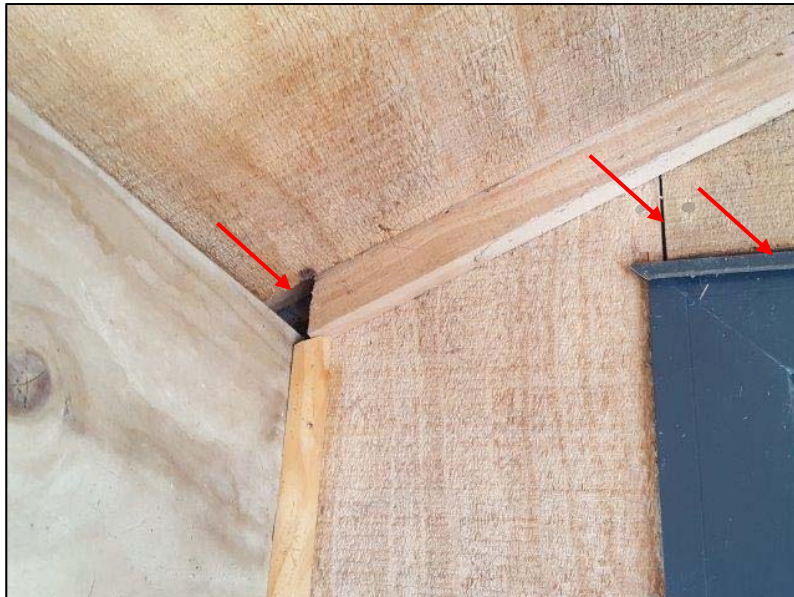
Photo 83: Head flashing is installed over sleepout door. No trim is installed over vertical junction above head flashing. End of soffit trim is poorly finished, leaving gap at beam junction
