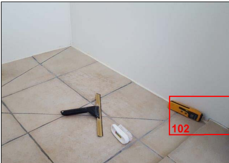
Photo 101: Seratone or similar wet wall linings in master bedroom ensuite shower are reliant on a sealant bead for waterproofing. The current manufacturer's instructions for tiled installations indicate a fully sealed junction between the two materials above a tiled upstand, which allows for drainage off the wall linings. Refer indicated closeup in following photo
