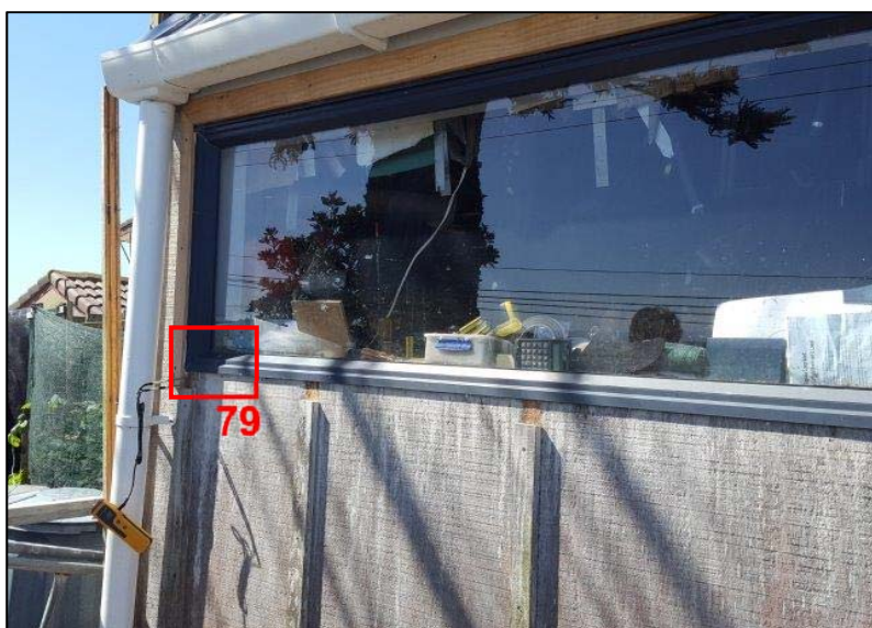
Photo 78: Workshop window with sill trim removed. Refer moisture testing in next photo
