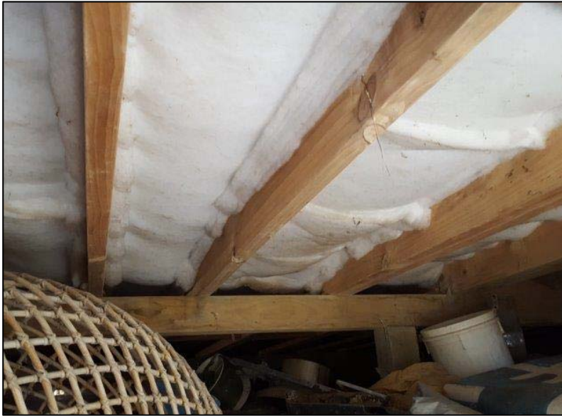
Photo 100: Polyester type insulation appears to be well installed between floor joists with no visible gaps
