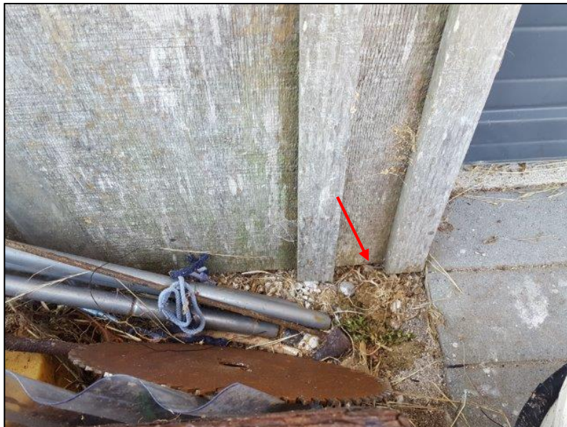
Photo 35: Cladding adjacent to garage door is in contact with unfinished ground. Refer Dodd drawings for planned remediation (Minor Alterations 2) and photo 26 for location
