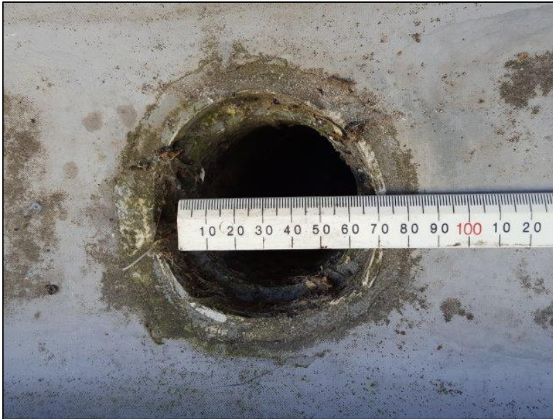
Photo 43: 65mm diameter deck outlet. No overflow is installed, but is not considered necessary, refer next photo
