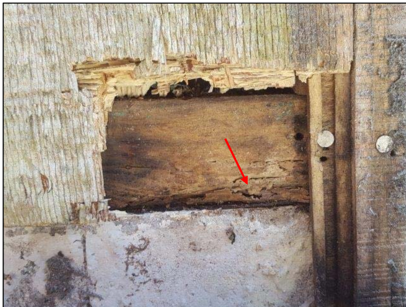
Photo 32: Visibly decayed bottom plate, garage NE elevation. Refer next photo
