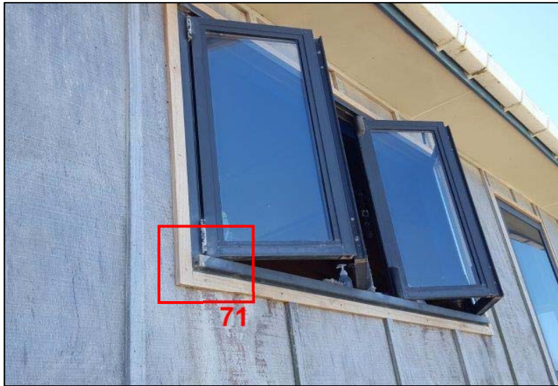
Photo 70: Bifold windows on SE elevation. Battens have recently been installed to all sides of some joinery. A photograph on page 90 of the Dodd cladding weathertightness report dated 17/12/15 indicated that sealant applied to a window jamb junction was in poor condition and the repair proposal recommended that all joinery should have cover battens installed to their perimeters. Refer to comments and photos below
