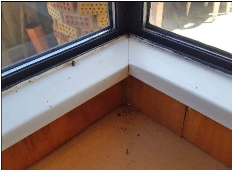
Photo 8: Interior view of seat below window junction. No indication of any moisture penetration to the interior
