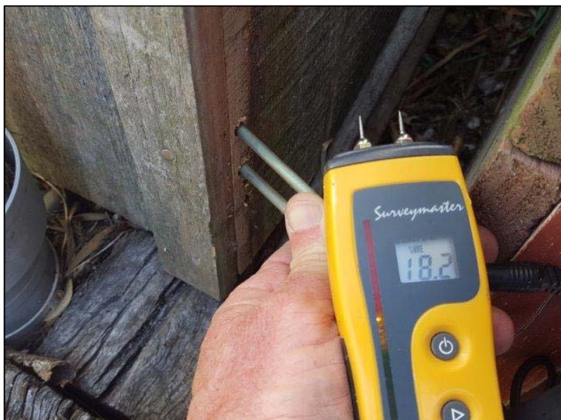
Photo 24: MC 18% slightly elevated moisture reading at west corner of garage. Ground clearance is less than 225mm required to meet Acceptable Solution. Refer Dodd drawings (Minor Alterations 2)
