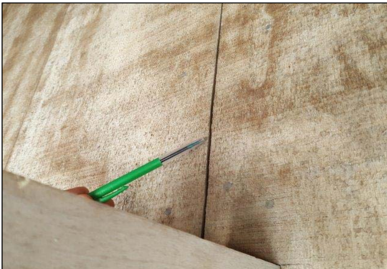
Photo 89: No trim installed over butted plywood cladding junction
