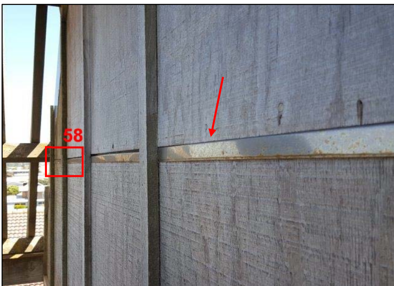
Photo 57: The plywood cladding is finished hard down on the metal horizontal flashings in some locations, which does not comply with the manufacturer's instructions. Also refer next photo
