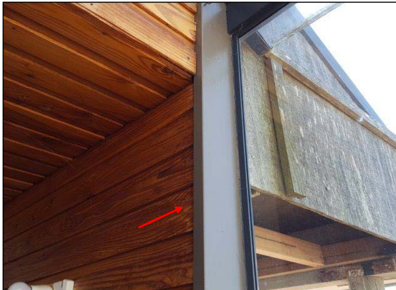
Photo 4: View of bulkhead from bathroom interior. No indication of any moisture penetration to the interior walls below the bulkhead was noted. Cladding below the bulkhead will need to be removed to check for any wall damage below
