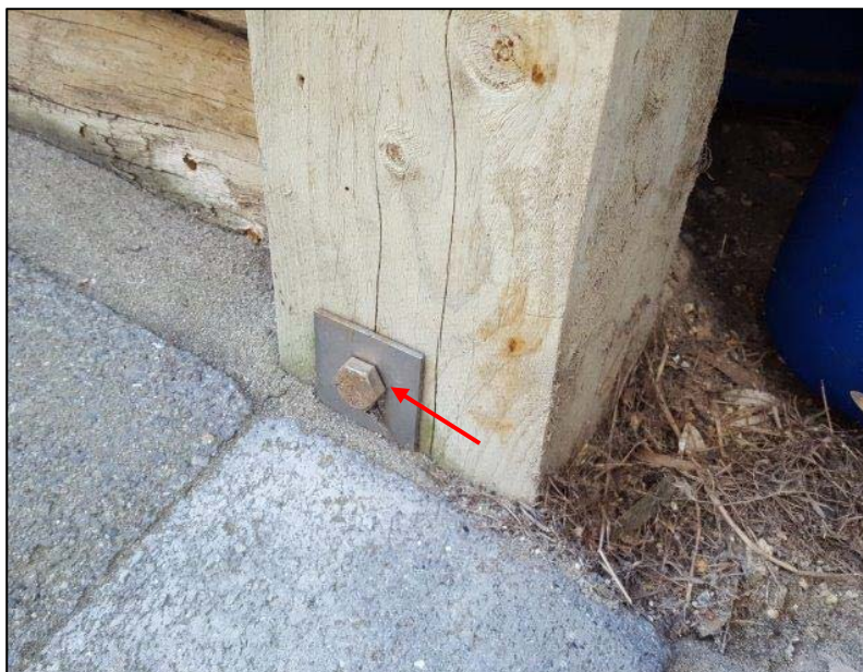
Photo 99: Stainless steel bolted connection
