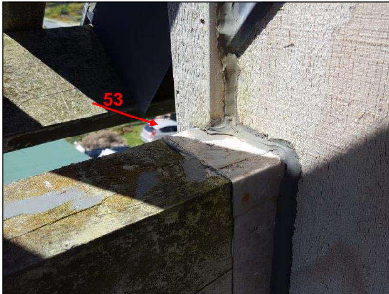
Photo 52: Vulnerable cladding penetration junction at east corner of master bedroom (typical). Refer next photo for view of other side of junction. Refer Dodd drawings for planned remediation (Minor Alterations 5)
