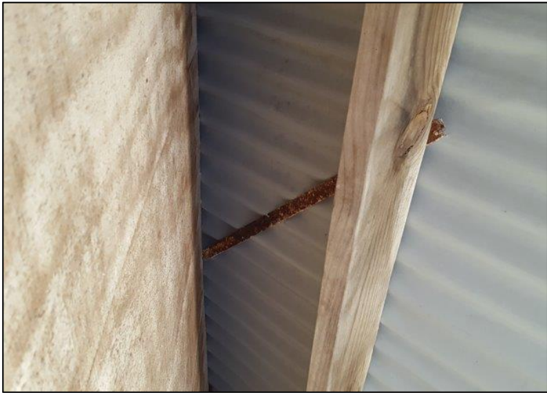
Photo 95: Corrosion on sleepout roof strap bracing above deck needs attending to
