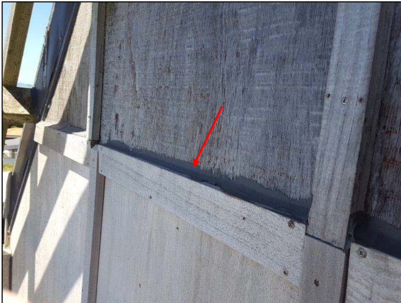
Photo 59: Horizontal flashing on NE beach elevation has been battened and partially sealed. It is unclear whether the sealant was added as a preventative measure or if the cladding was leaking. Also refer next photo and photo 50 for location
