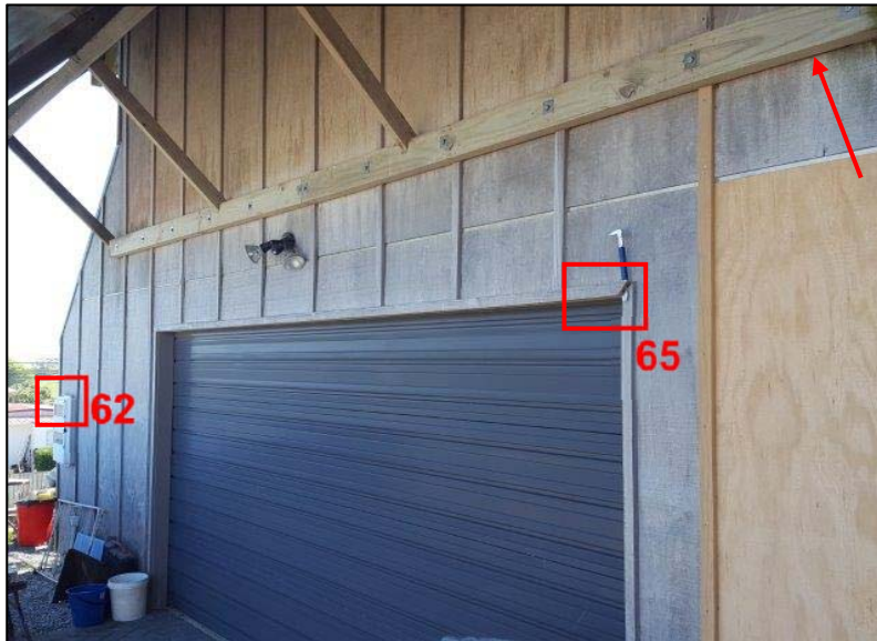
Photo 64: SE garage elevation. Pergola (indicated) has been spaced off cladding. Refer head flashing closeup in next photo, and general elevation on photo 26
