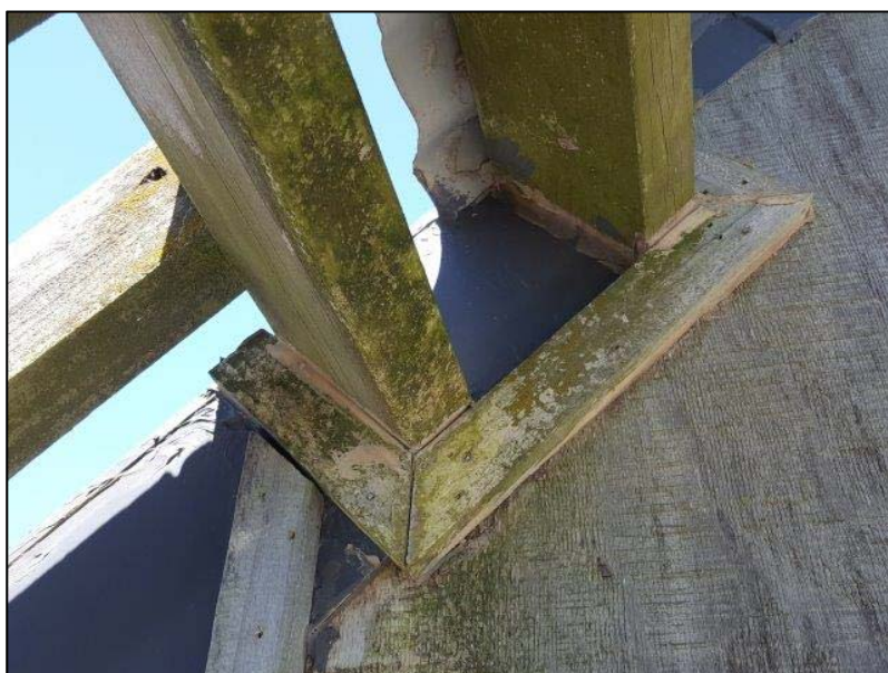
Photo 54: Vulnerable double cladding penetration junctions above master bedroom. Refer Dodd drawings for planned remediation (Minor Alterations 5)
