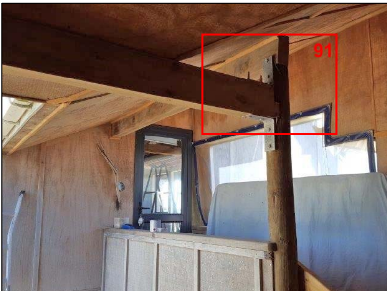
Photo 90: Pole and beam junction in entry area between house and garage. Refer indicated closeups in following photos
