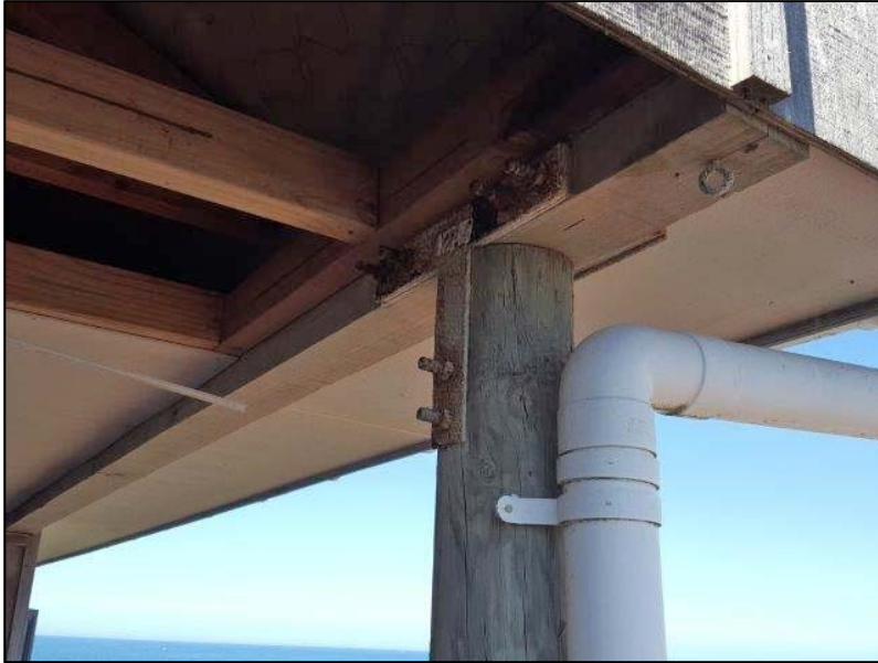
Photo 94: Corrosion to structural connection in laundry soffit area on SE elevation needs attending to. There is some inconsistency with a mix of stainless steel and galvanised connections/bolts installed. Refer photo 1 for general location
