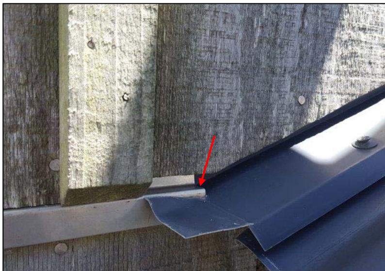
Photo 38: End of apron flashing terminates behind horizontal flashing. No kickout flashing is installed. Refer Dodd drawings for planned remediation (Minor Alterations 3)
