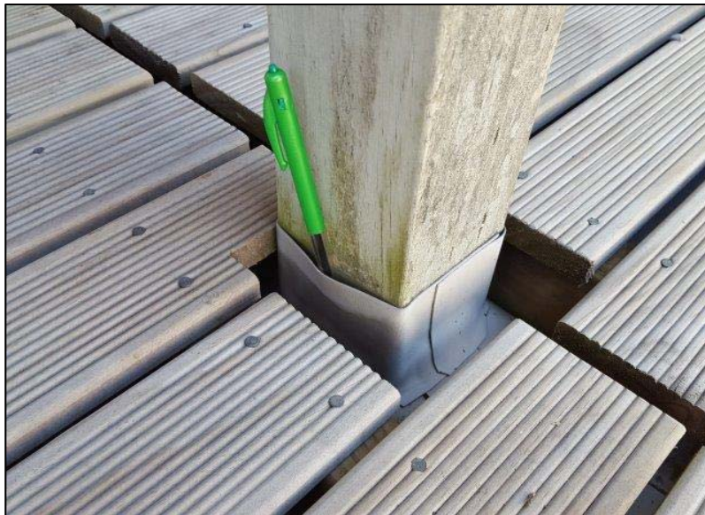
Photo 41: Unsealed butyl rubber turnup at verandah post. Refer Dodd drawings for planned remediation (Minor Alterations 4). Refer following photo with floating decking lifted
