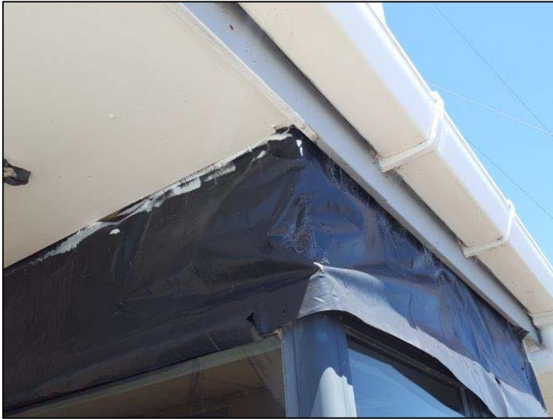
Photo 7: Cladding removed above north boxed window (by others). Refer to Dodd drawings for planned remediation (Repair No. 2)
