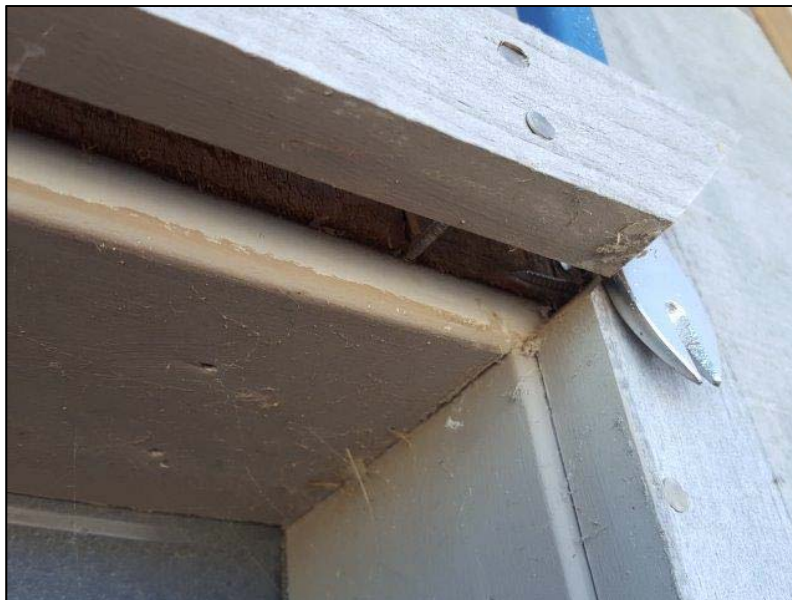
Photo 65: No head flashing has been installed to garage door head. Not considered a weathertightness risk with wide canopy protection overhead
