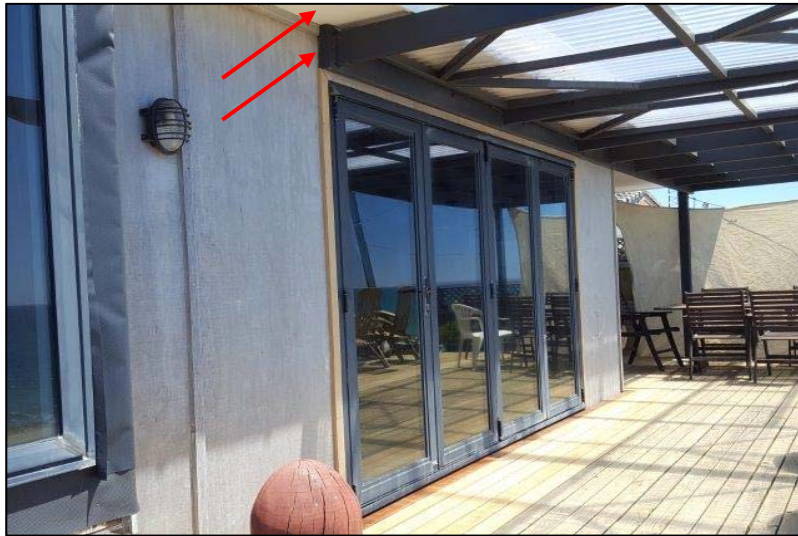
Photo 25: Pergola on NE elevation has been spaced off cladding as per Dodd drawings (Minor Alterations 1). 550mm eaves protection (including gutter) is provided on the NE elevation (except where reduced by the boxed window projections)
