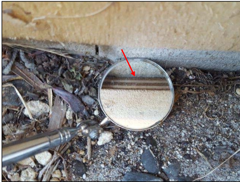
Photo 28: New cladding is fixed hard against garage slab. Dodd drawings specified existing framing to be straightened and packed out if required to provide 6mm clearance between cladding and concrete slab of garage. Note the cladding appears to be generally clear of the concrete slab elsewhere on the garage and workshop. Refer following photos
