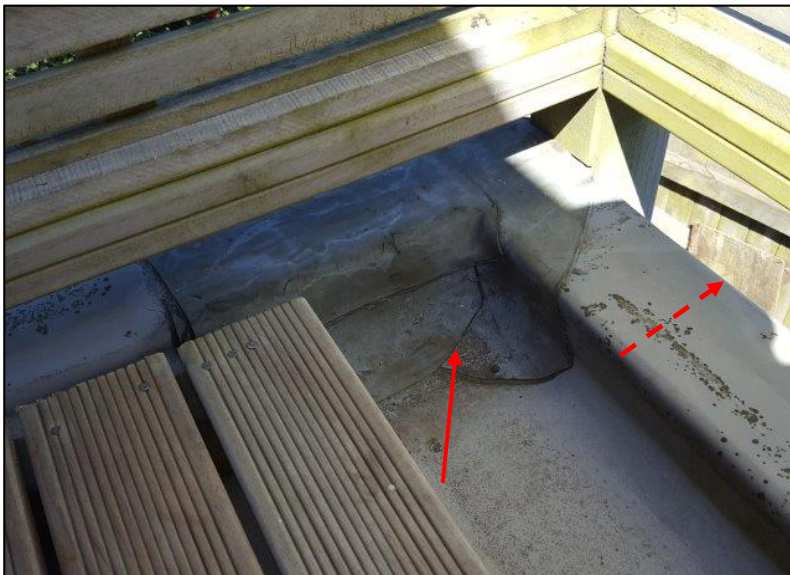
Photo 44: Butyl rubber deck cladding appears to be reasonably well detailed at west corner. No overflow is installed, but is not considered necessary, as any overrun will be to the exterior over the fully waterproofed nib upstands
