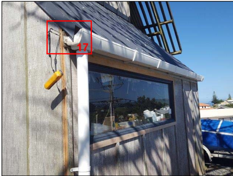
Photo 16: External corner junction with cover batten removed at top plate, west corner of workshop. Refer following photos
