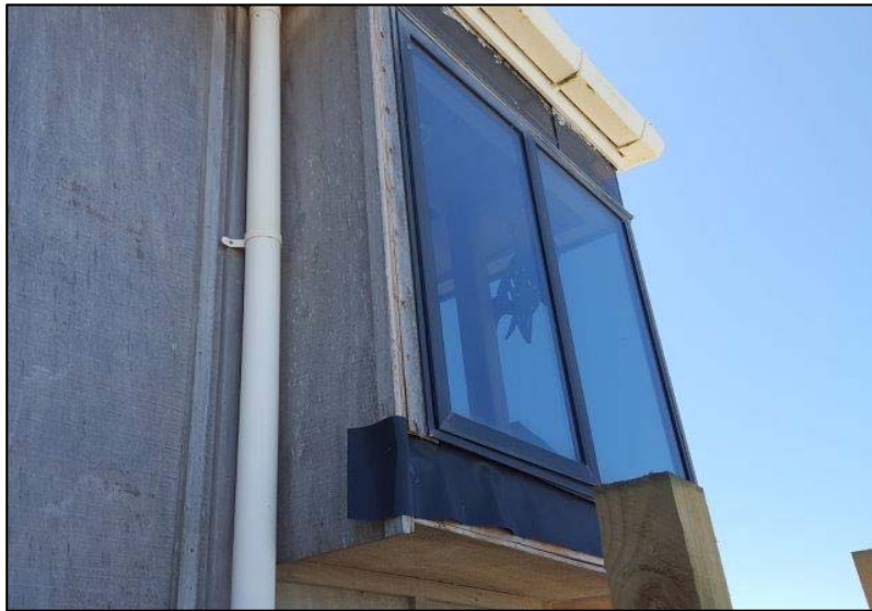
Photo 10: East boxed window (SE elevation, cladding removed by others). Refer to Dodd drawings for planned remediation (Repair No. 2)
