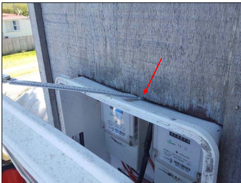
Photo 63: No flashings installed around meter box – rule penetrates into workshop
