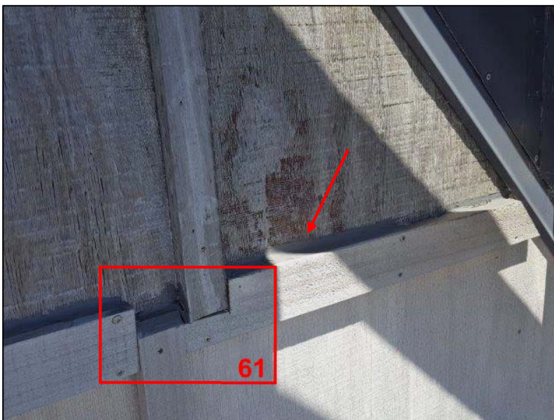
Photo 60: Horizontal flashing on NE beach elevation has been battened. Refer closeup in next photo and photo 50 for location
