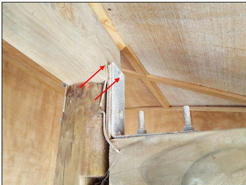
Photo 92: Top beam connection to timber pole is reliant on a single bolted connection and four wire dogs, all in the end and lower third of the beam. The connection could be improved significantly by installing a longer bracket with double bolted connection to the top beam. Refer next photo at other end of the single bolted connection
