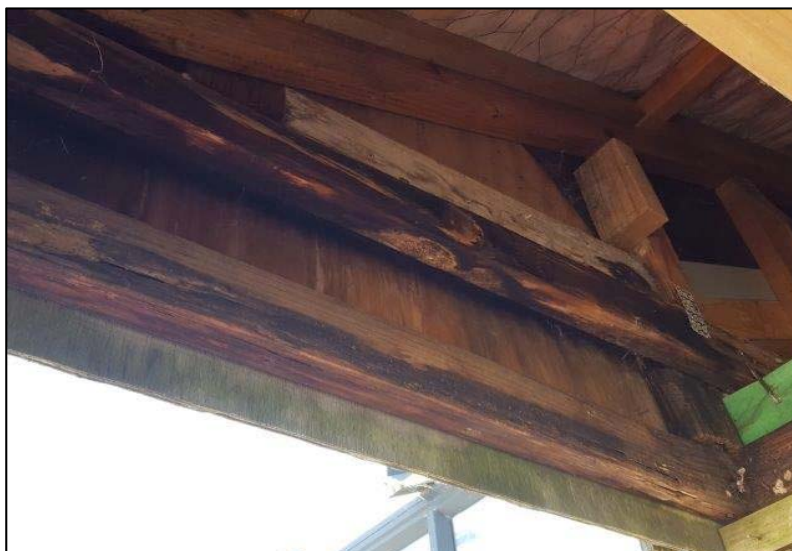
Photo 3: Damaged bulkhead framing. Refer to Dodd report investigation photos 9-13 and Dodd drawings for planned remediation (Repair No. 1)
