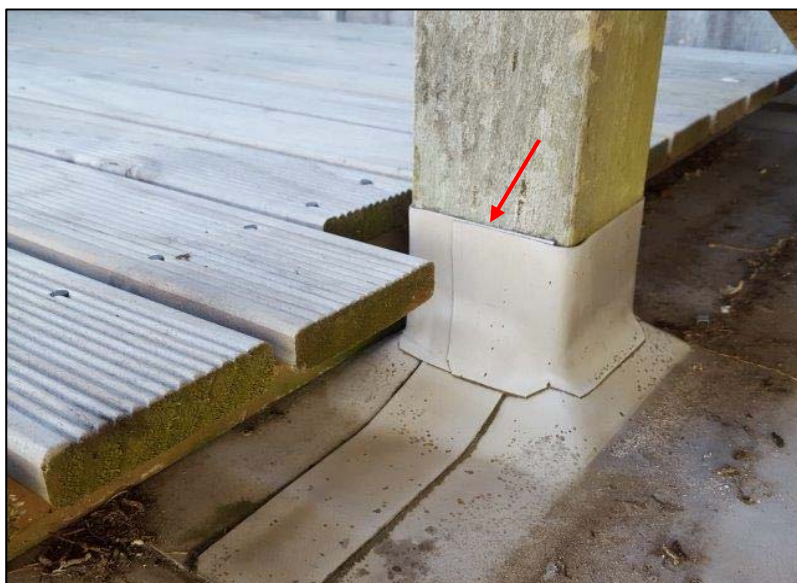
Photo 42: Butyl deck cladding appears to be reasonably well detailed apart from the unsealed turnup
