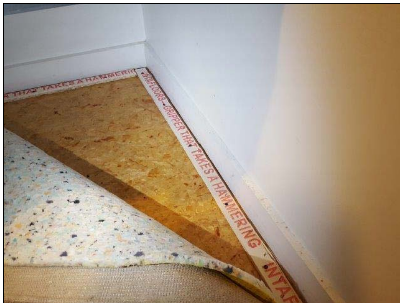
Photo 104: Strand flooring adjacent to shower in immaculate condition. Any leakage from the shower would rapidly indicate as staining on the flooring. The flooring adjacent to the shower in the master bedroom was also immaculate, indicating that the shower waterproofing is performing adequately
