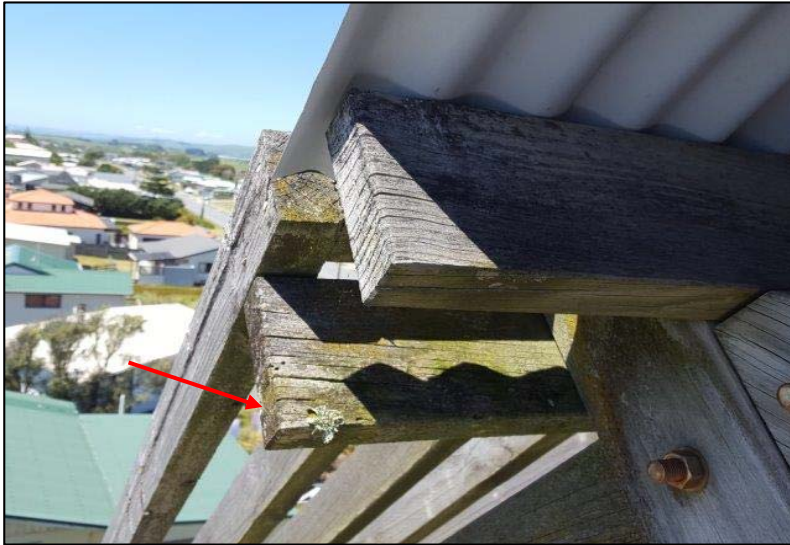
Photo 55: Exposed ends of beams are weathered and appear to have not been maintained. Builder mentioned that the pergola type beams may be replaced with roofing, which would provide improved weather protection to the cladding. Stainless steel bolts are in good condition (with minor staining only visible in photo)
