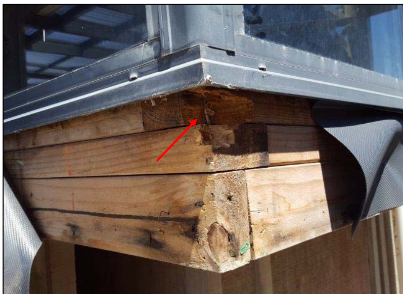
Photo 6: Visibly decayed timber framing below north boxed window (cladding removed by others). Cause of failure may be related to lack of external corner moulds (refer photos 14, 18 & 20). Photographs on page 90 of the Dodd cladding weathertightness report dated 17/12/15 indicated that the timber cover battens (assumed in this location) were in poor condition. Refer to Dodd drawings for planned remediation (Repair No. 2)
