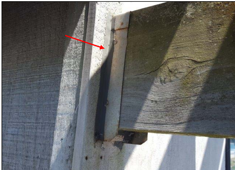
Photo 53: View of vulnerable beam penetration junction
