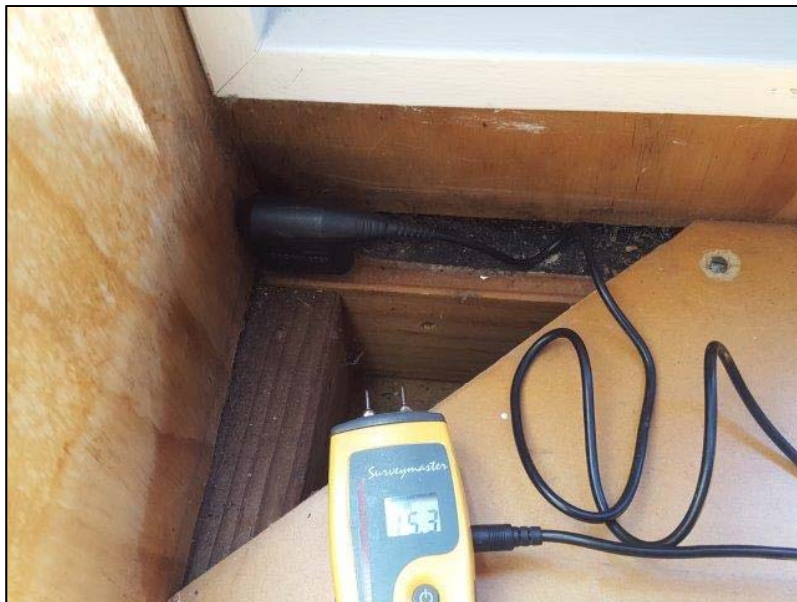
Photo 11: Interior view of seat below end of window, NE elevation. Corner of window seat has been cut out by others. Timber is waterstained, MC 15% currently normal moisture reading taken
