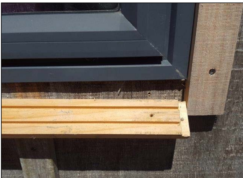
Photo 75: Grooved rear face of sill trim with ends rebated to allow drainage from grooves. Flat top surface allows water to pond on sill trim, potentially trapping water against the cladding and restricting drainage from behind the window flange. If sill trim is retained, the top 5mm of the trim needs to be removed to allow drainage from behind the window flange. The top surface of the trim also needs to be sloped 15° to prevent accumulation of water. Refer next photo for moisture test
