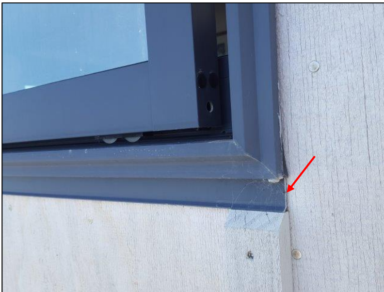
Photo 68: Sill flashing has been installed to master bedroom window
