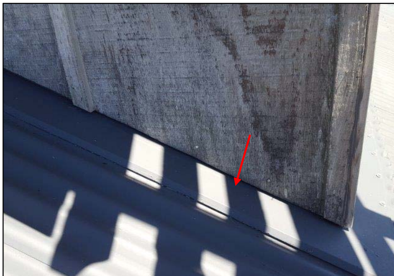
Photo 39: Minimal cladding clearance to apron flashing at upper east corner of house. Difficult to maintain bottom edge of cladding but unlikely to result in weathertightness failure within prescribed 15 year durability period
