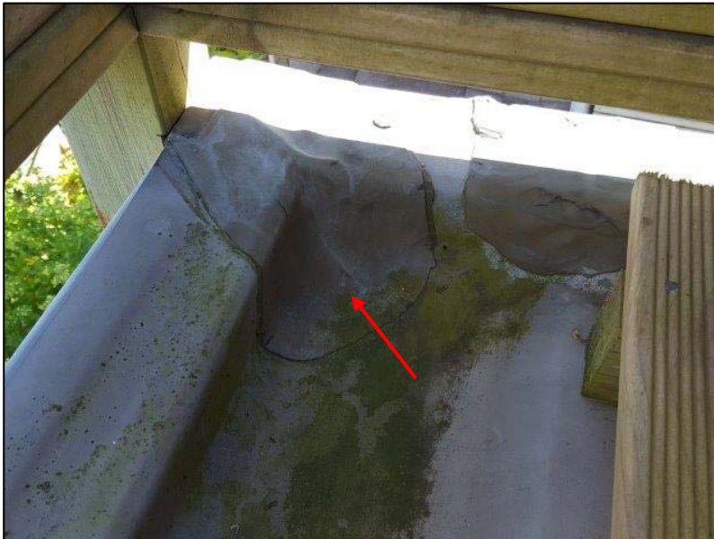
Photo 47: Butyl rubber deck cladding appears to be reasonably well detailed at north corner
