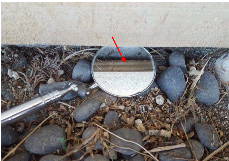
Photo 30: Adequate gap provided between cladding and concrete slab. Note ground clearances don't meet Acceptable Solution
