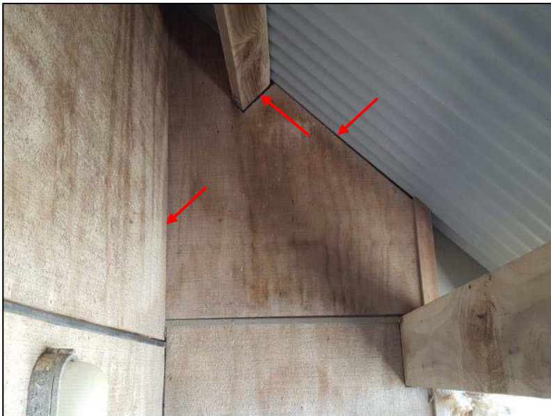
Photo 86: Sleepout deck end wall. No trims are installed to internal corner and cladding junctions to beam and roof
