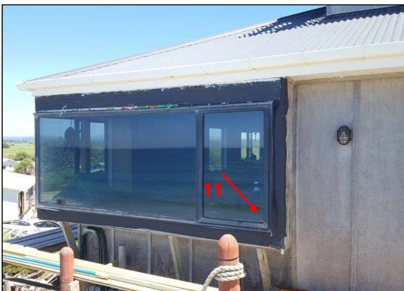
Photo 9: East boxed window (NE elevation, cladding removed by others). Refer to Dodd drawings for planned remediation (Repair No. 2)
