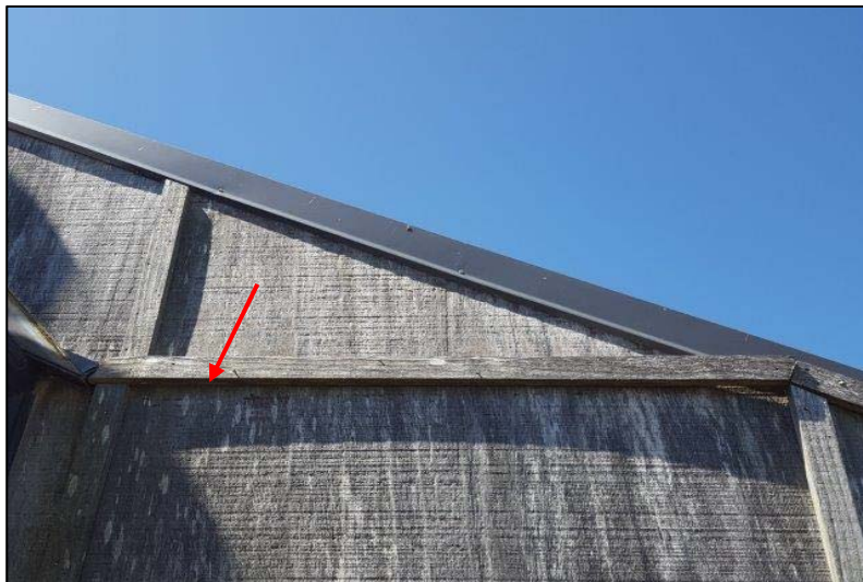
Photo 2: Laundry bulkhead on SW elevation. The plywood cladding has been poorly installed, with the lower cladding sitting proud of the upper cladding, allowing water penetration, refer next photo for view inside bulkhead
