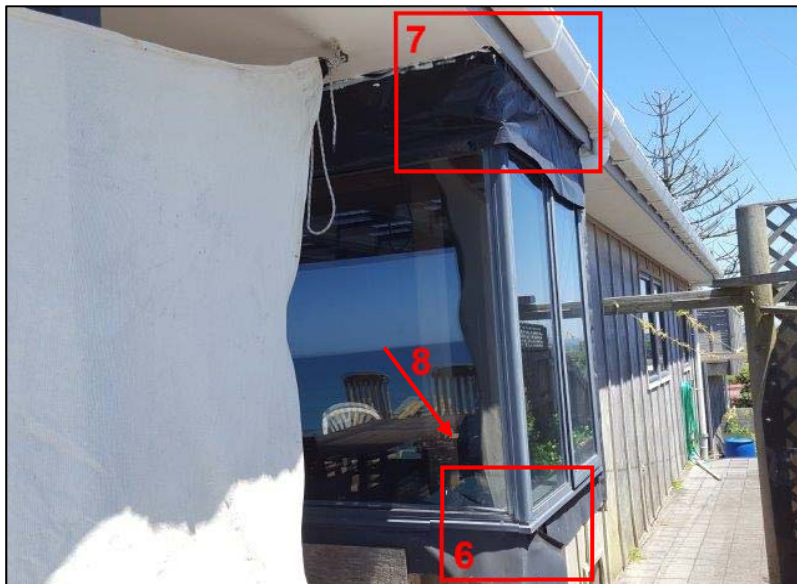
Photo 5: North boxed window (cladding removed by others). Locations of following photos indicated
