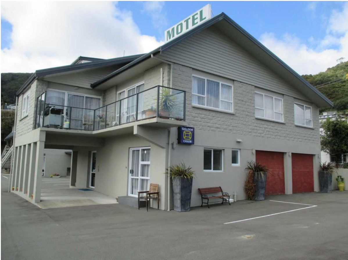
West and North side
