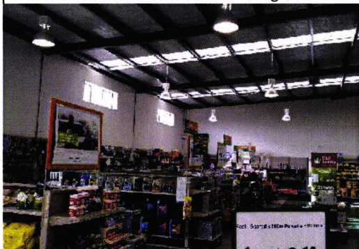
Mono sloped roof - rafters and purlins supporting roof
