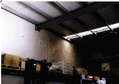
Frames attached to concrete panel walls & roof bracing
