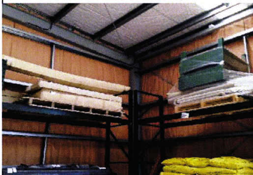
Roof and wall bracing
