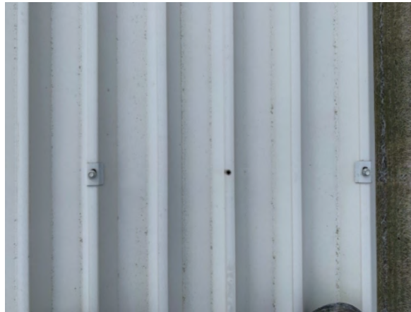
Missing fixing
