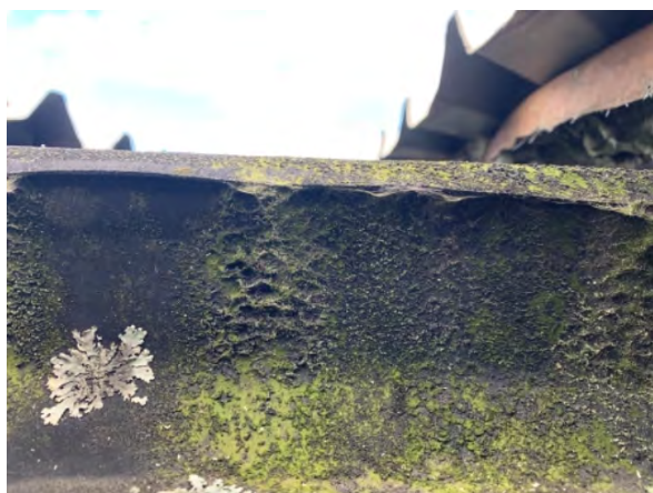
Lifting lap in gutter
