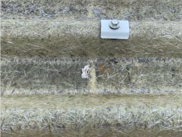
Sealant repair done to skylight
