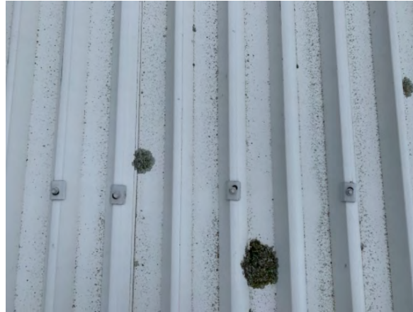
Screws with split neo washers
