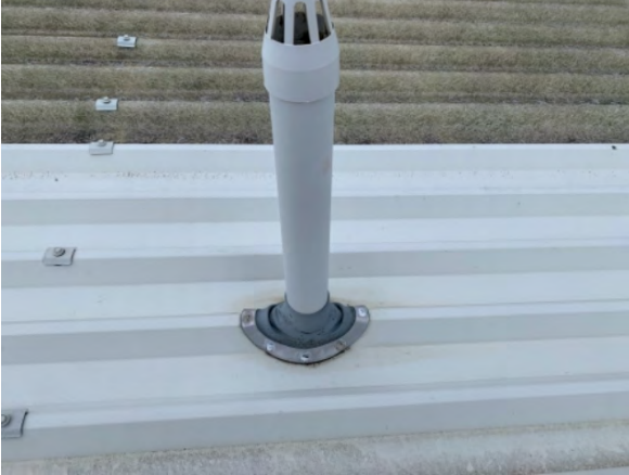
Dektite and vent penetration
