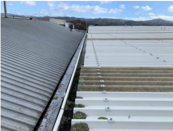
Box gutter overview
