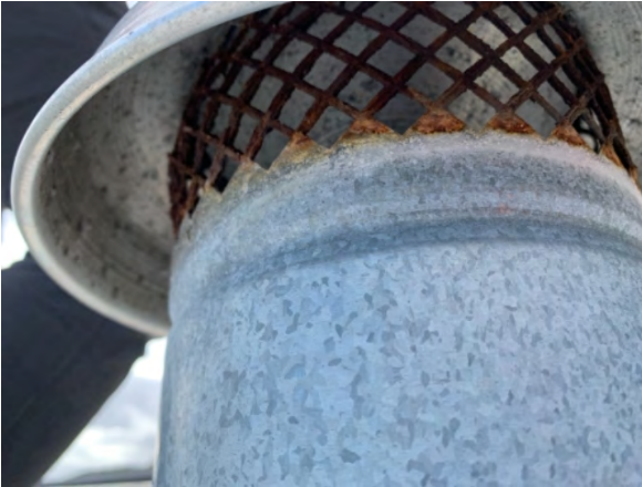
Corroded cowls
