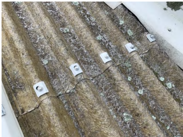
Skylight lap area where two skylight sheets lap
