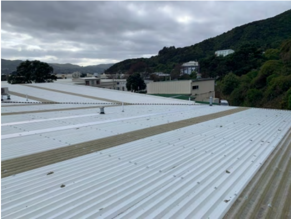
Roof over view
