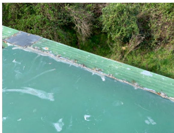
Faded sealant
