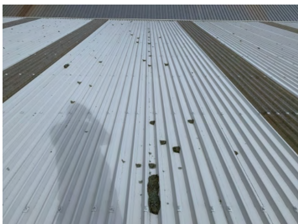
Moss on metalsheets Overview of moss present on sheets
