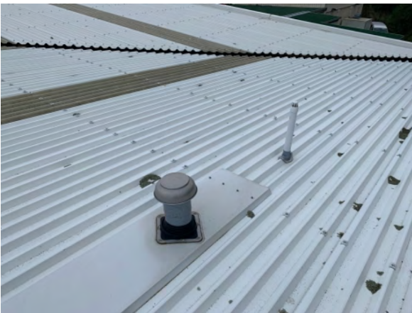
Penetrations covered by a tray flashing.
