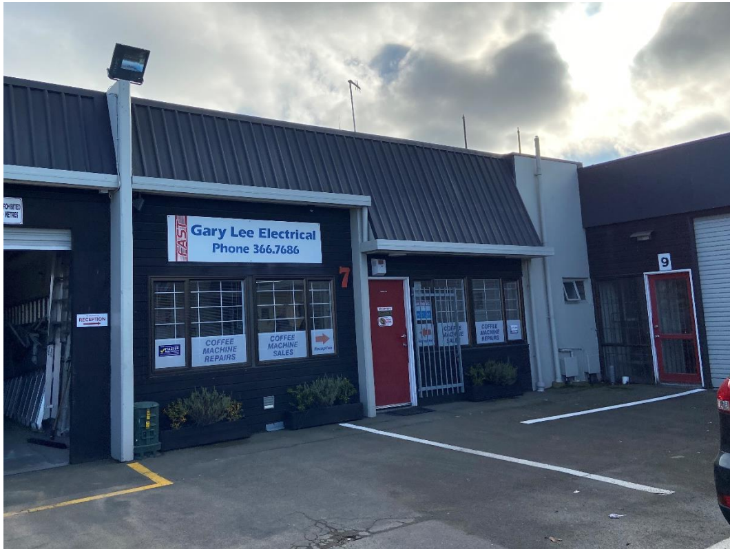
Photo C 1 – Front façade (unit 7)
