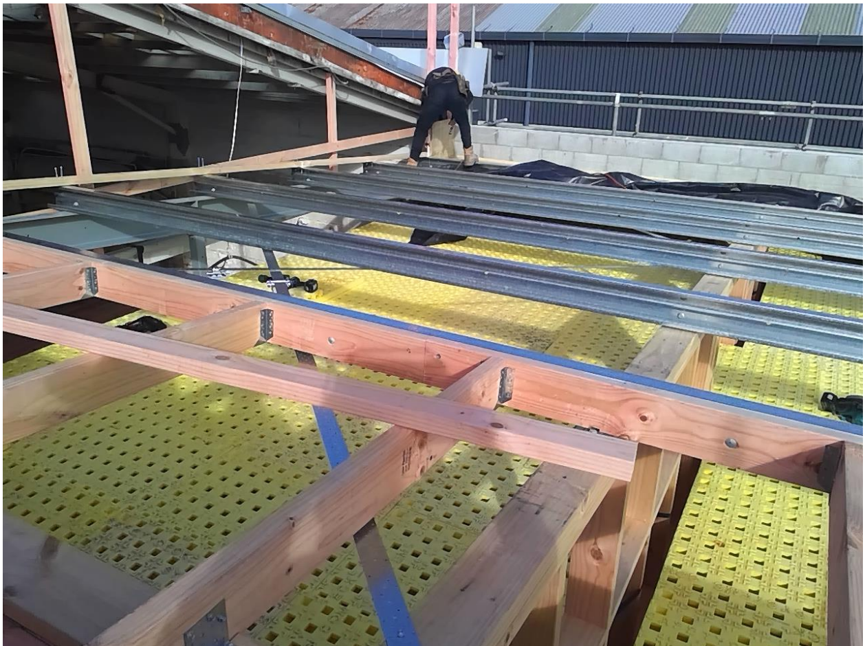
roof plane brace
