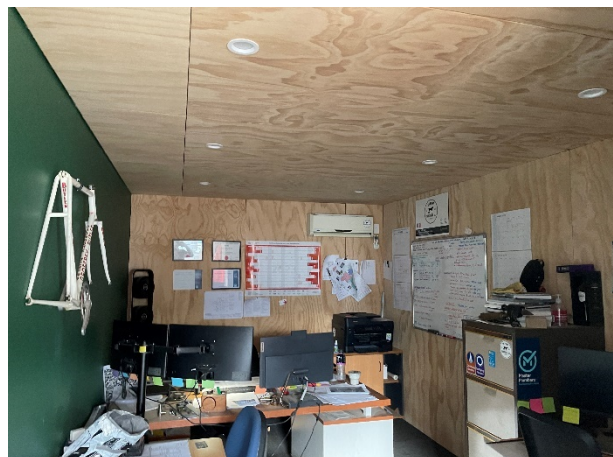
Photo 6: Typical Timber Framing Extension Including Plywood Ceiling.
