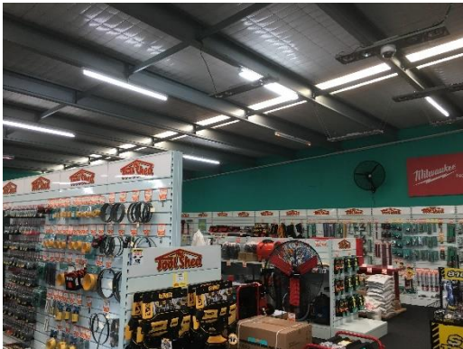
Photo 3 – Steel roof framing for interior of Unit 33 – Tool Shed
