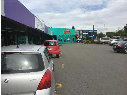
Photo 1 – Front units towards street – Building 2 looking to Unit 33
