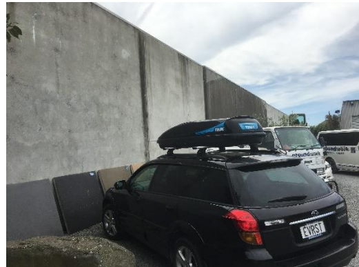
Photo 4 – Rear of building 2 showing concrete wall from original building in Unit 31
