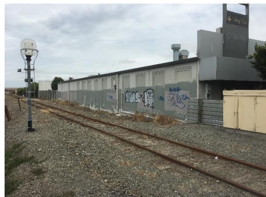
Photo 6 – Rear concrete walls at Building 1
