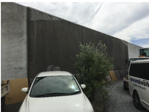
Photo 5 – Original wall for Building 2 in Unit 31
