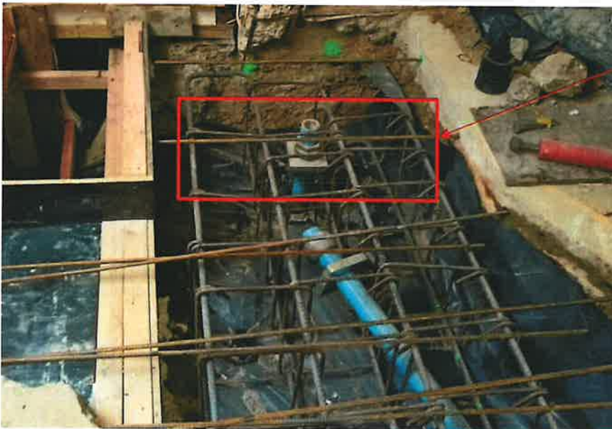
Figure 5. Concrete beam at grid D
