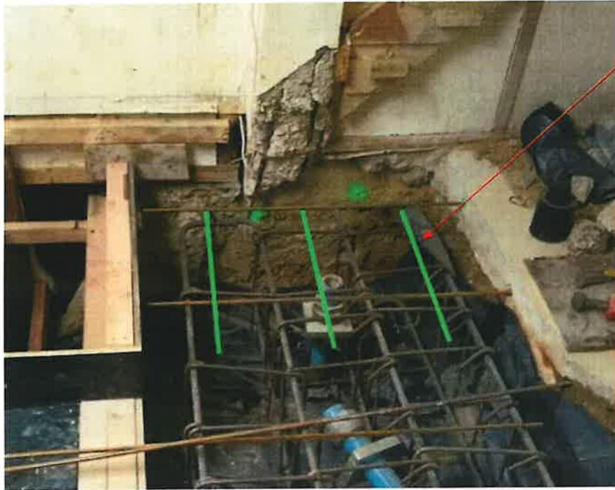
Figure 6. Concrete beam at grid D
