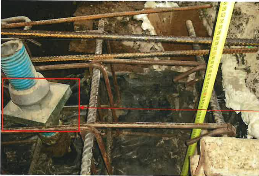
Figure 4. Concrete beam at grid D
