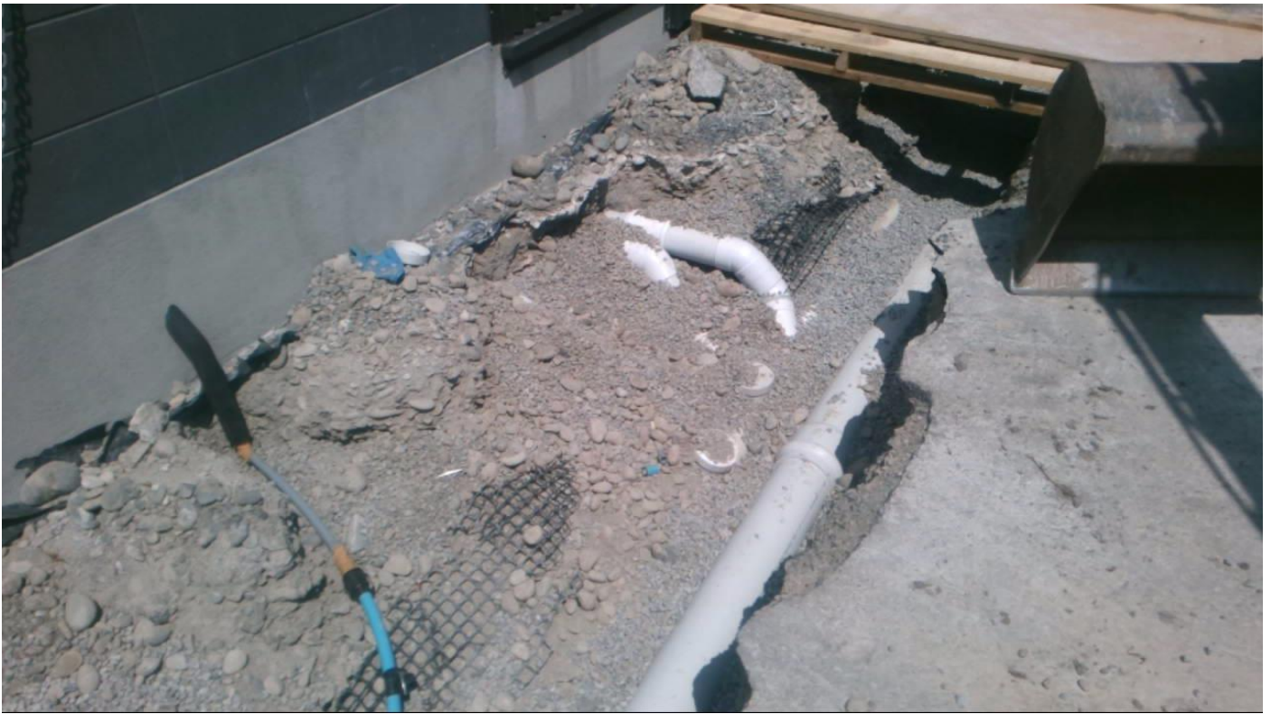
sewer vent and wc Taken at 11:42 AM on Tuesday 26/11/2019
