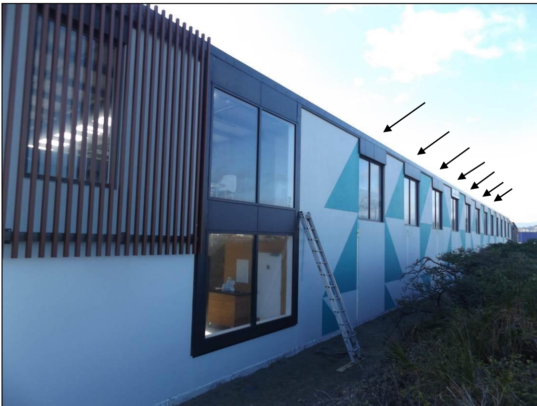
The southern elevation – showing the painted fibre-cement panels that act as the head covers for the windows below
