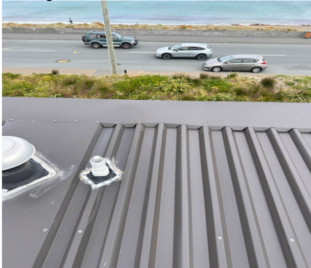
Evidence of poorly applied sealant
