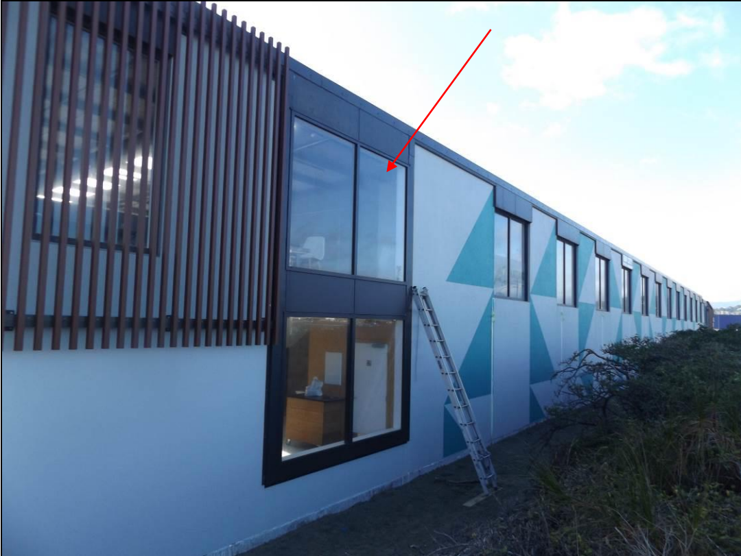
The large southern elevation western corner feature window assembly - Unit 35
