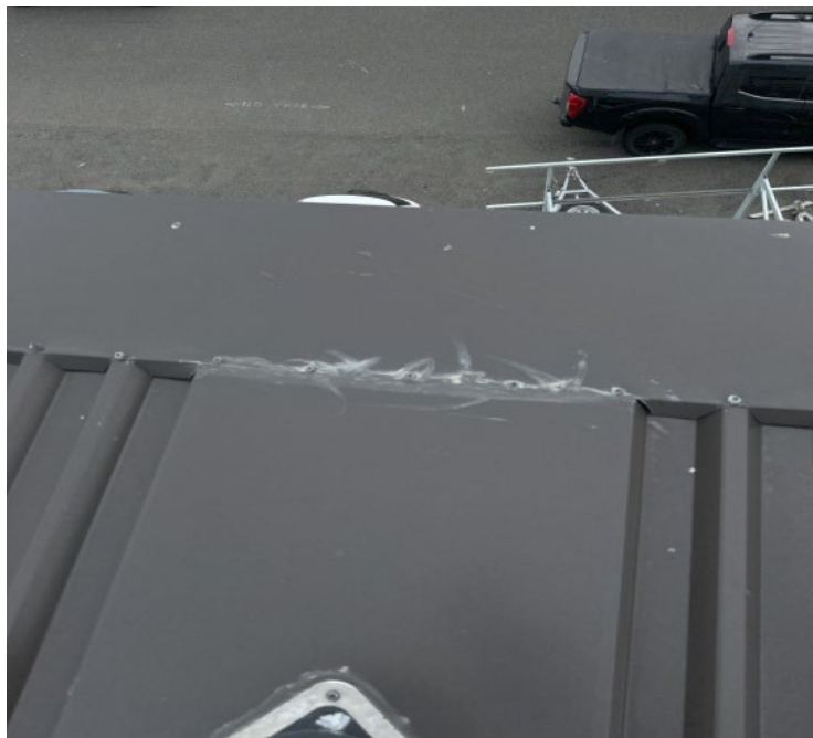
Evidence of poorly applied sealant
