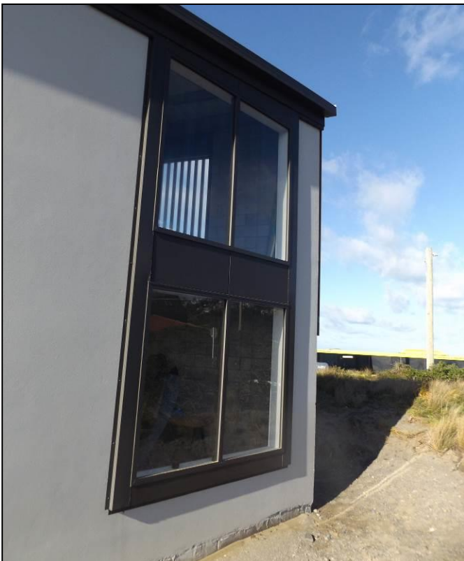
The western large western corner window assembly – Unit 35
