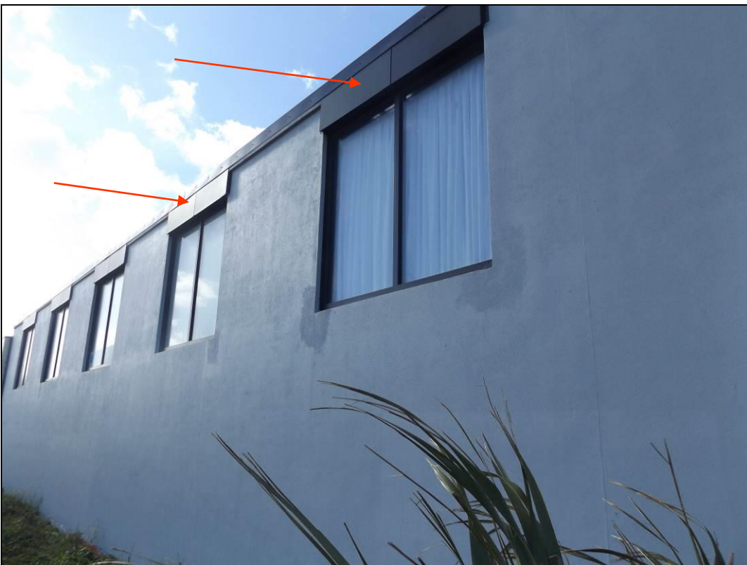
Showing the western elevation fibre-cement panels
