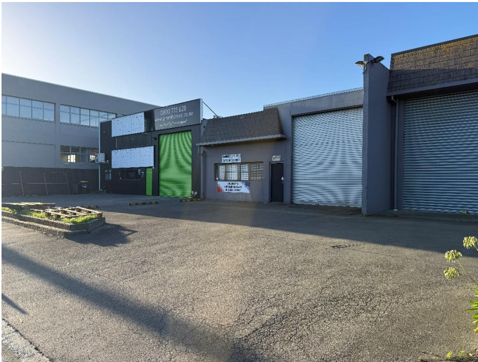
Site from Essex Street
