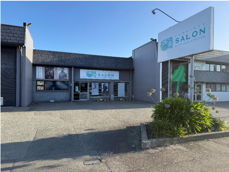
Site from Cashel Street
