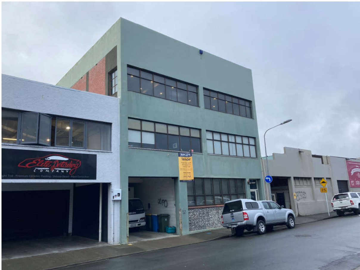
Figure 2: View of building from Hania Street looking southeast.
