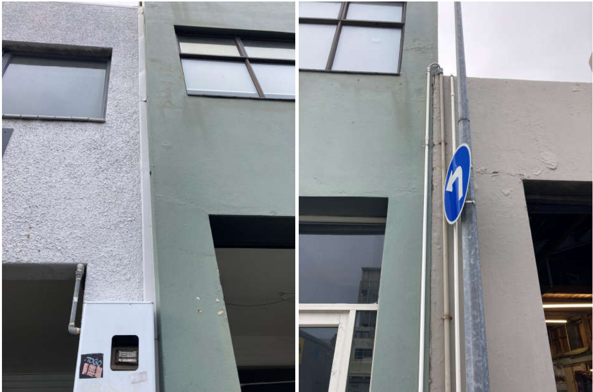
Figure 3: Adjacent Buildings to the North [above left] and to the South [above right].
