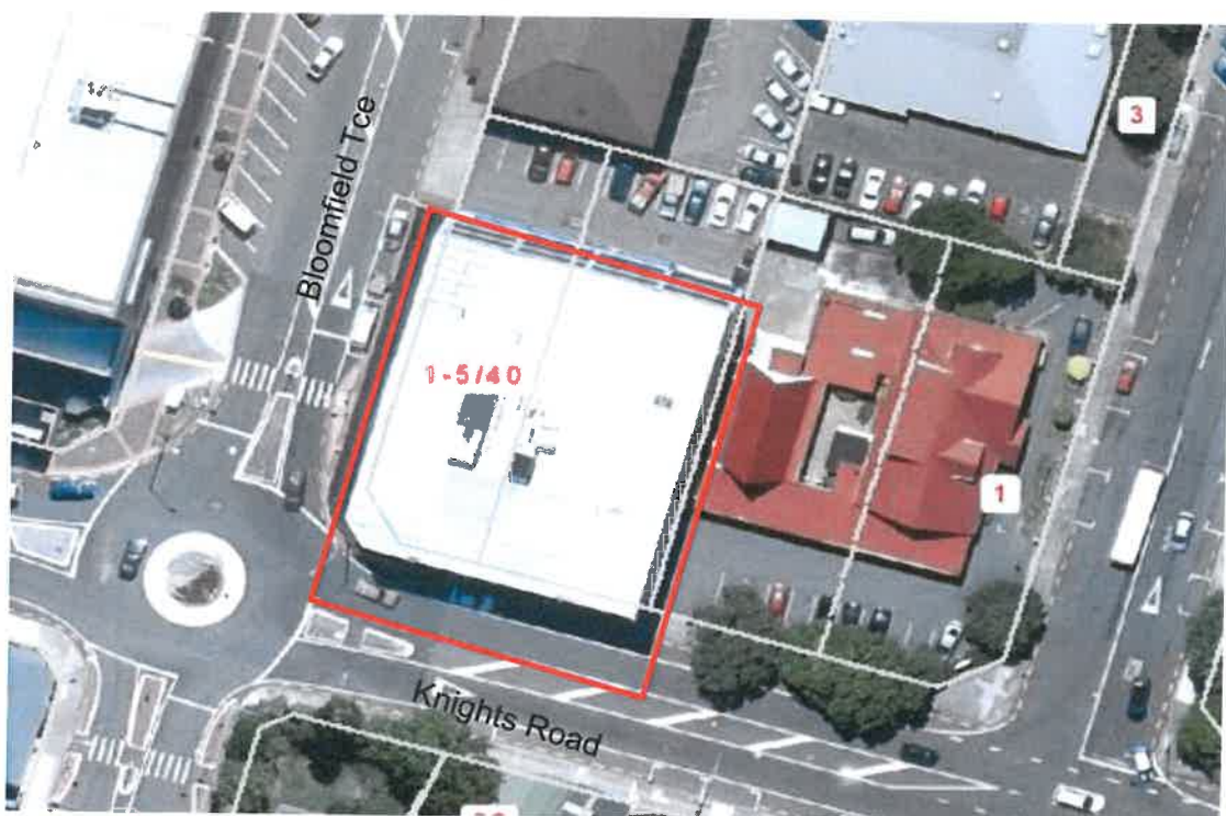
Photo 1: Aerial Photo of Woburn House at 44-45 Bloomfield Terrace, Lower Hutt
