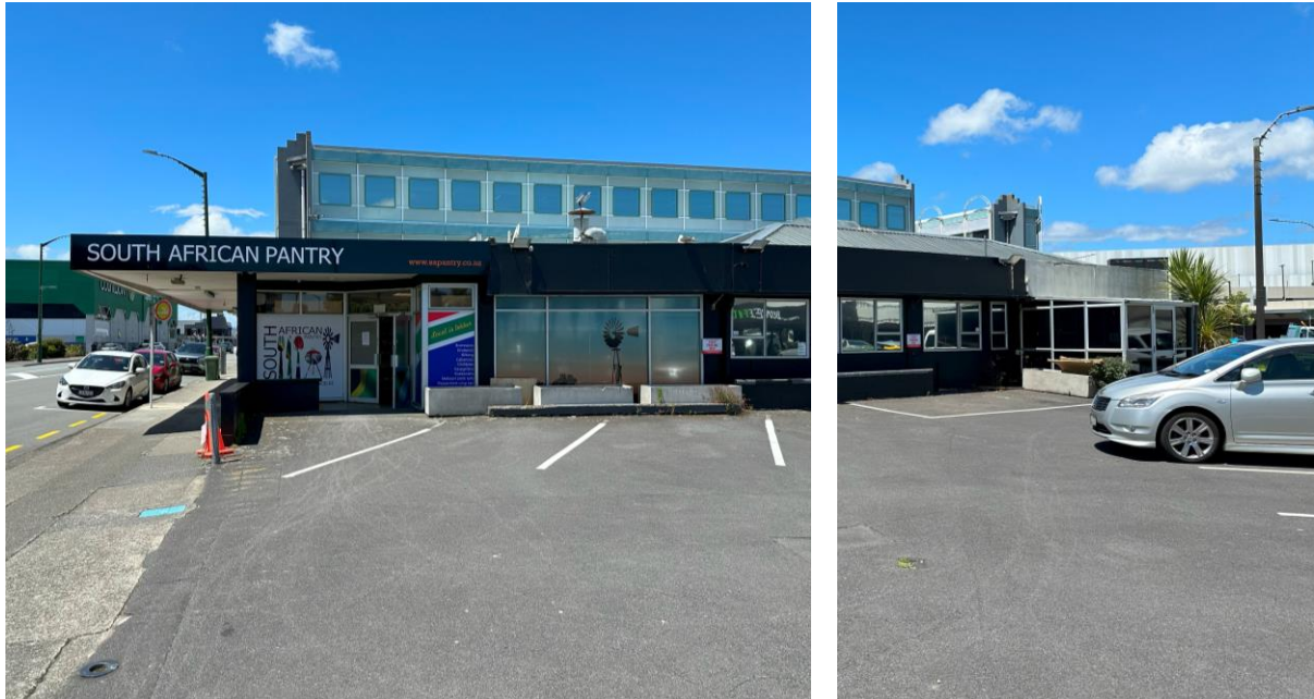
Figure 2.2: Elevation of the building from the south.
