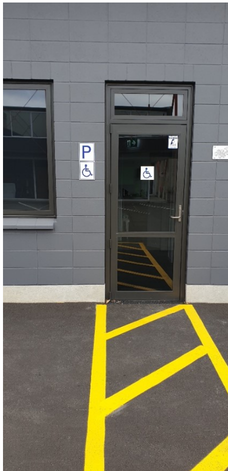
ISA sign installed
