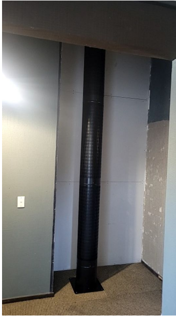
Floor penetration considered. Taken at 3:40 PM on Wednesday 9/04/2025
