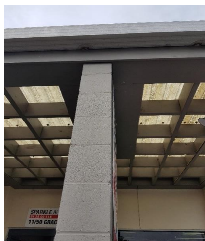
Figure 22: The overhang roof on the Western facade is in satisfactory condition but would benefit from a wash.
