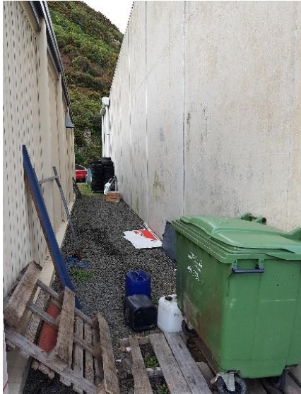
Figure 26: Rubbish between the Central and Northern block.
