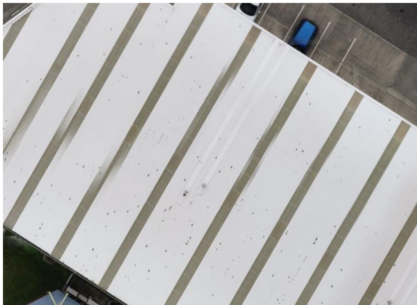
Figure 6: The Southern block roof with some visible lichen growth.
