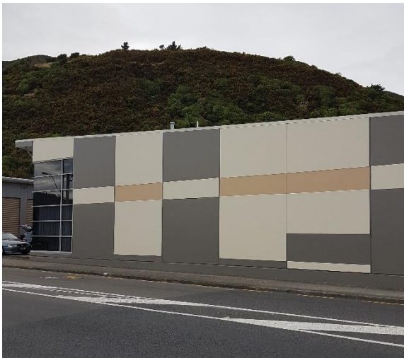
Figure 10: Paint in excellent condition on the Western facade.
