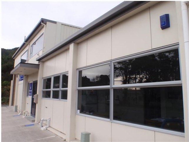
Figure 28: Single glazed aluminium framed window on the West Façade. Windows are in good condition and were detailed well during construction.
